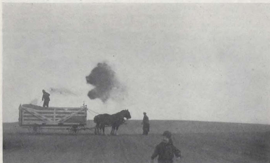
Spreading straw to control soil drifting on knolls.
