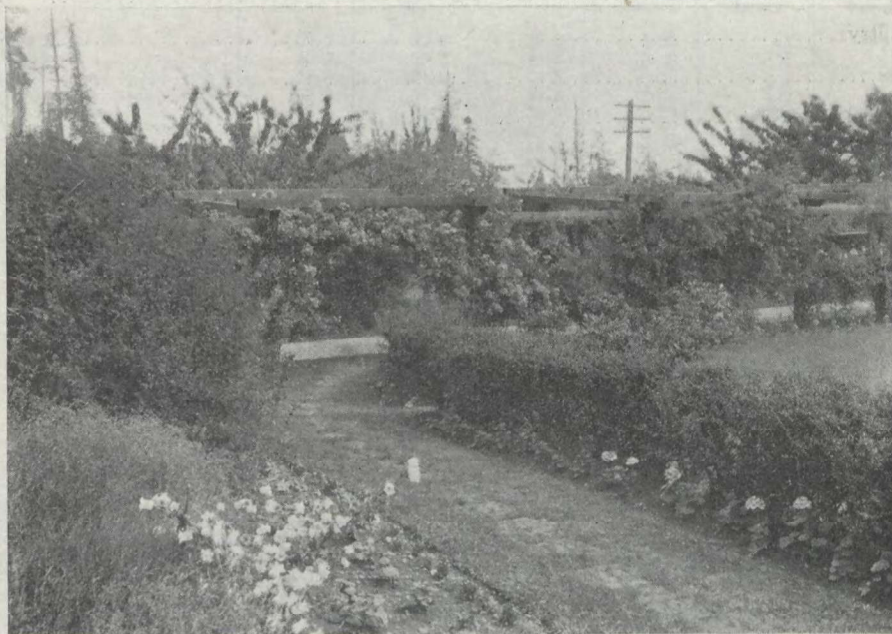
Entrance to the superintendent's house.
