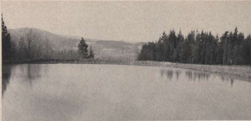
FIG. 6. Typical dugout on Saanich Peninsula. Capacity approximately 945,000 gallons.
