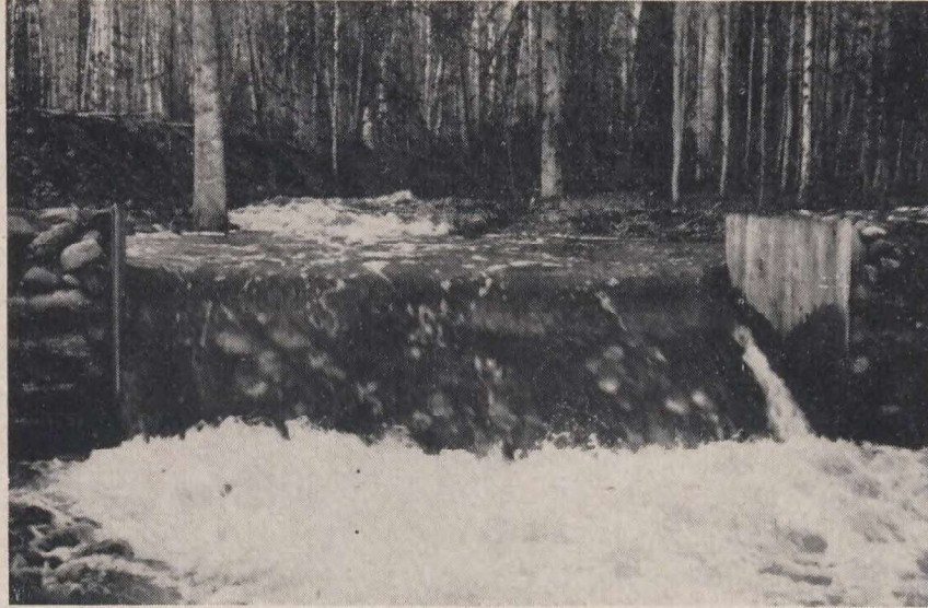
Fig. 2.—The weir constructed on Watching Creek to aid in recording runoff from timber range.
