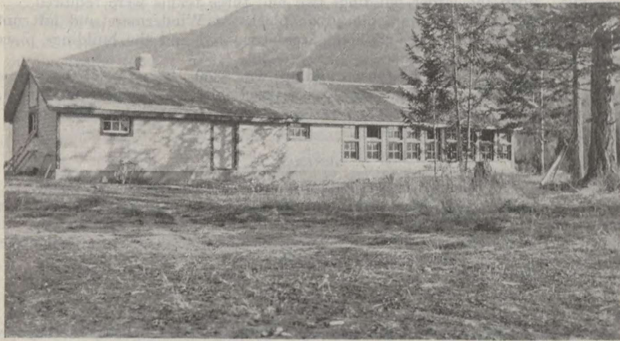
Combination poultry building including incubator-room, feed-room, record-room and three brooder-rooms.
