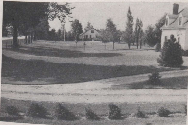
View of Grounds and Office on the Delhi Substation
