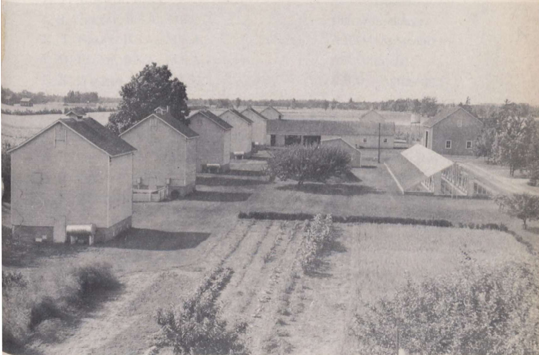
View of the kilns, implement shed, greenhouse and pack barn at the Experimental Station, Delhi, Ont.
