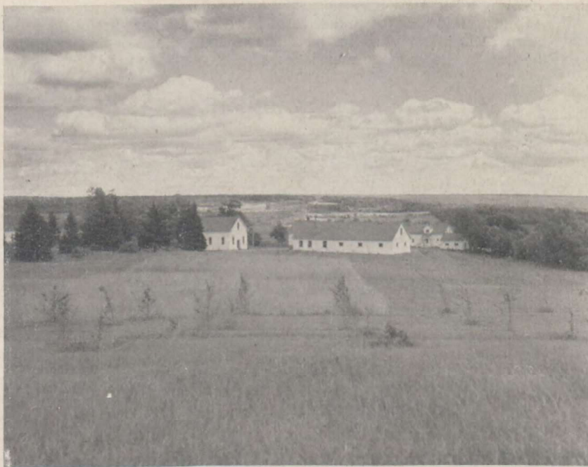
View of buildings, McDonald's Corner Substation—1951. Apple seedlings in foreground
