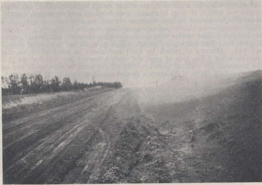
Effect of soil drifting. Dust bank filling road ditch on May 15, 1931. Loam swept off field shown in the illustration on page 27. Photo by Superintendent.
