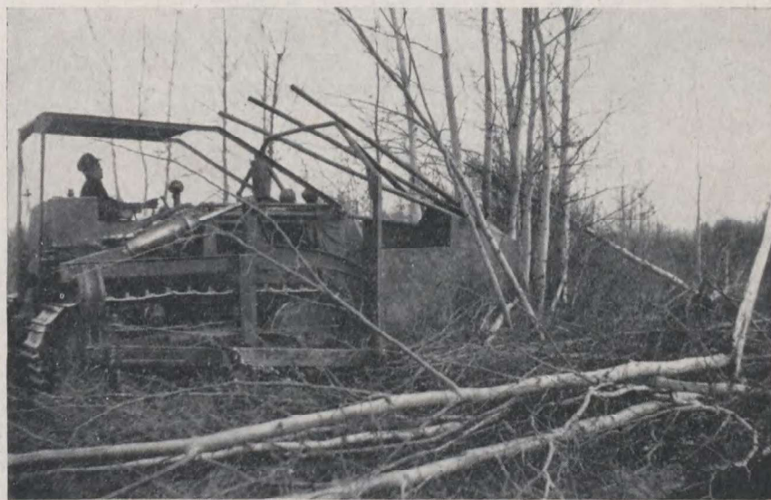
FIG. 50.—Brush cutting equipment at work, Baldonnel Station.
