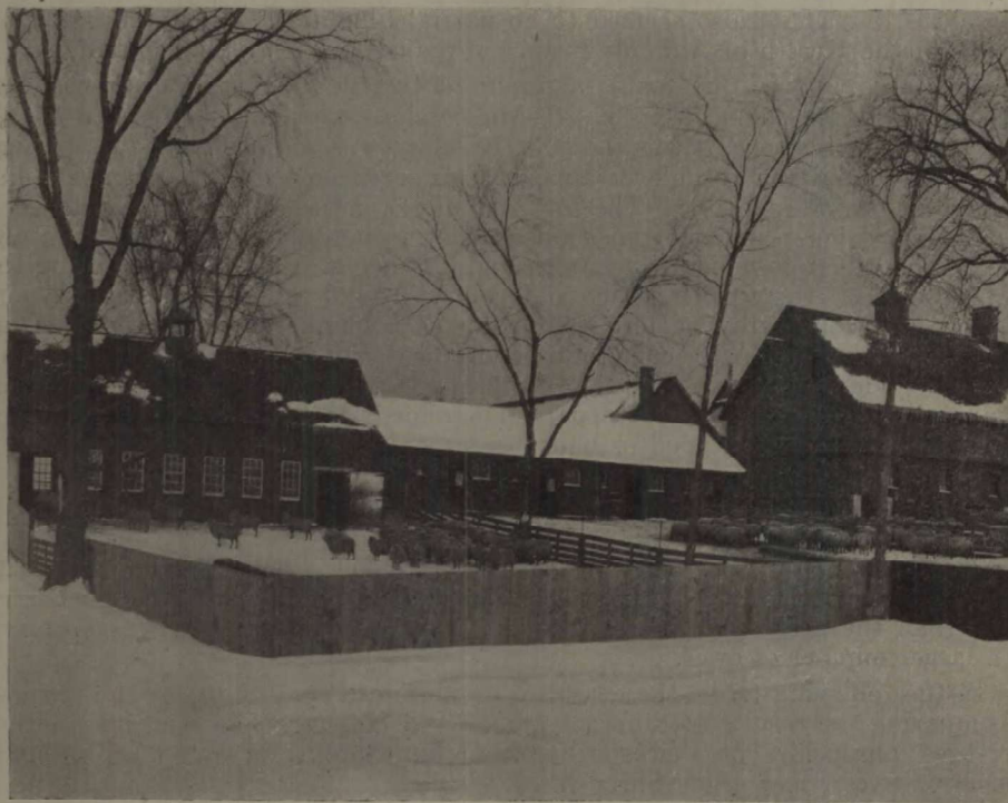
A general view of the sheep barns and paddocks after the rearrangement of the buildings, C.E.F., Ottawa.
