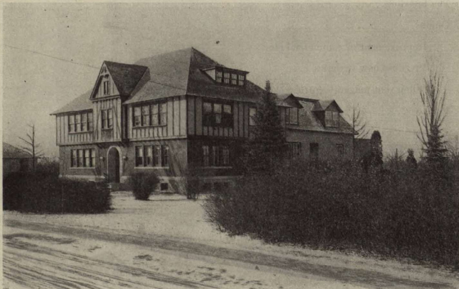
New Horticultural Building, Central Experimental Farm, Ottawa. (Photo by Frank T. Shutt)
