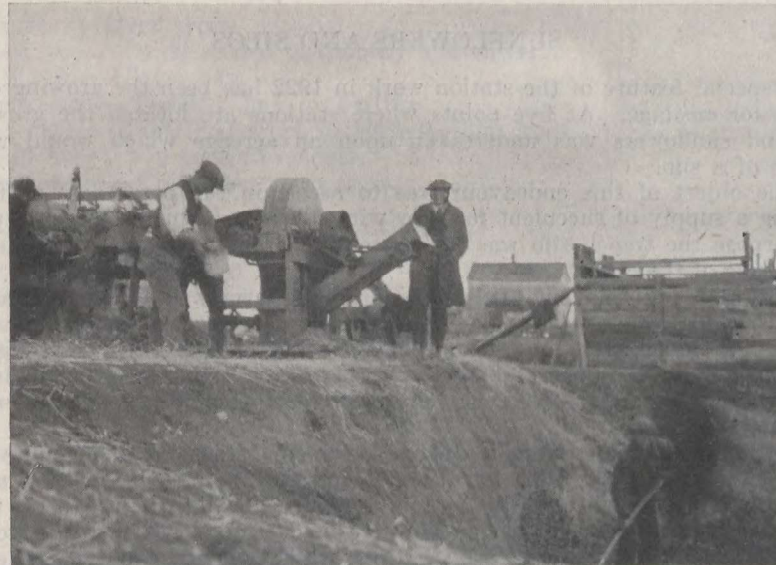
Showing plain cutting box with short carrier for delivery over trench, at Grassy Lake.
