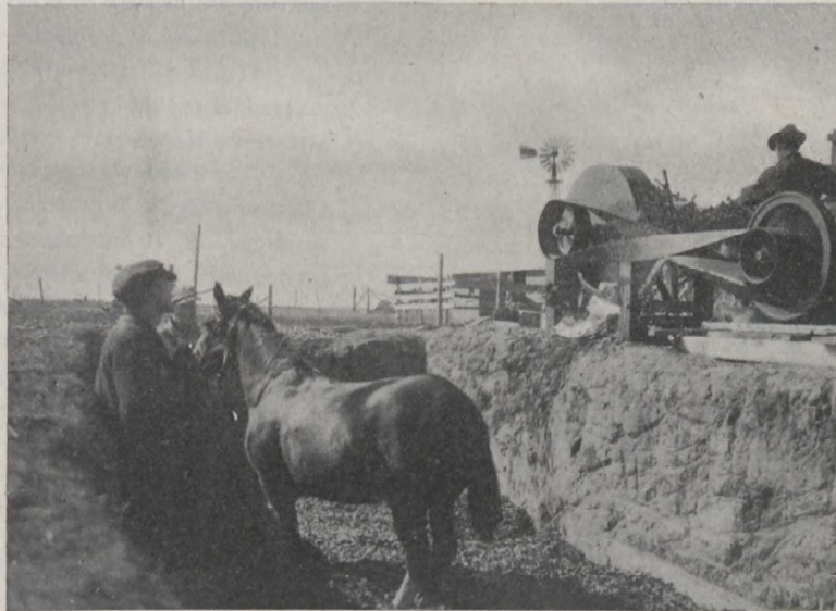
Filling trench silo with horse tramping cut material at Youngstown, Alta.
