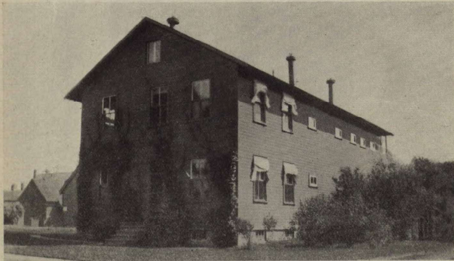
Main Office, Laboratory and Warehouse Building of the Tobacco Division, Central Experimental Farm, Ottawa, Canada.
