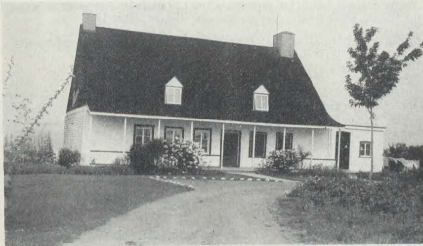
FIG. 24.—Farm Home, St. Pierre Illustration Station, 1947. This house is over 100 years old. The development of flower borders and the planting of hardy decorative shrubs is an important project.
