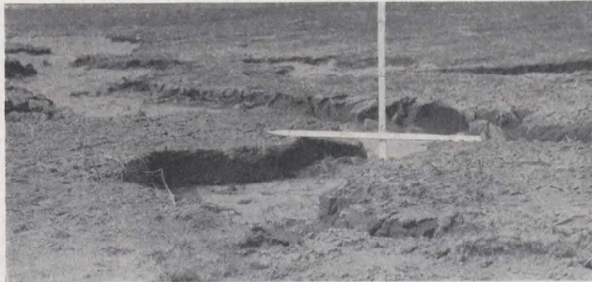
FIG. 7.—Gullying caused by run-off water. Erosion of this type can be levelled out by tillage but the top soil loss is irreplaceable.
