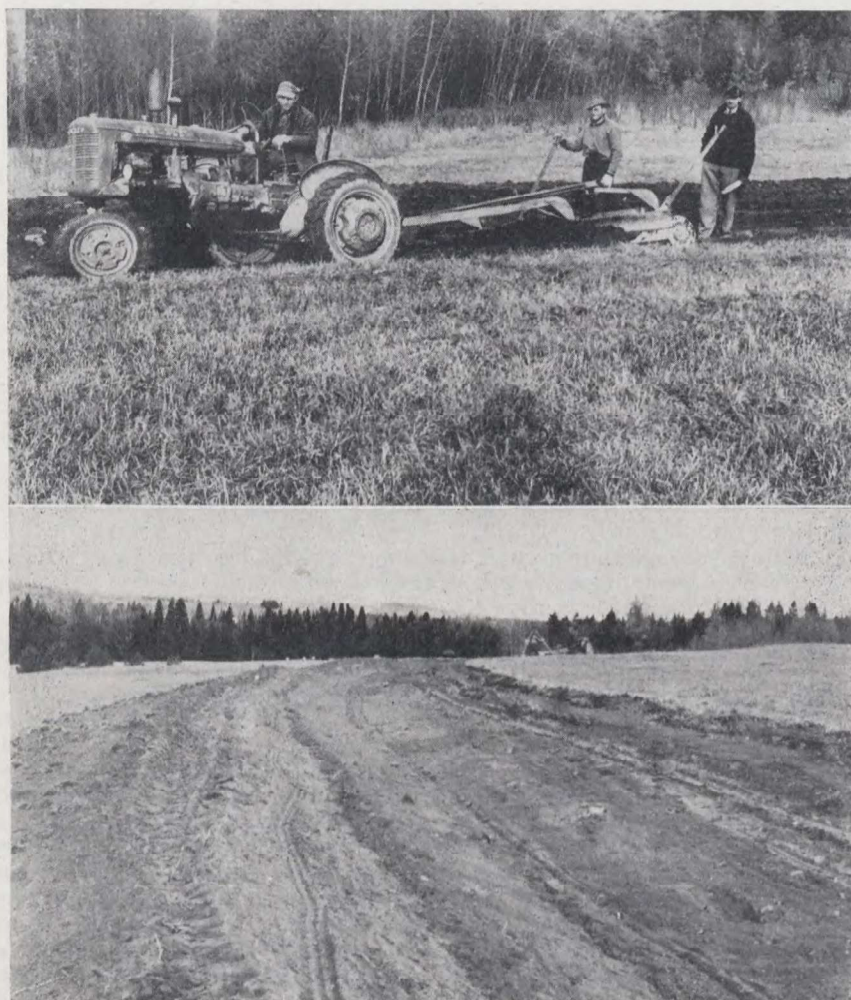
FIG. 8.—(Upper): Equipment used to construct diversion ditch, East Centreville Illustration Station.
