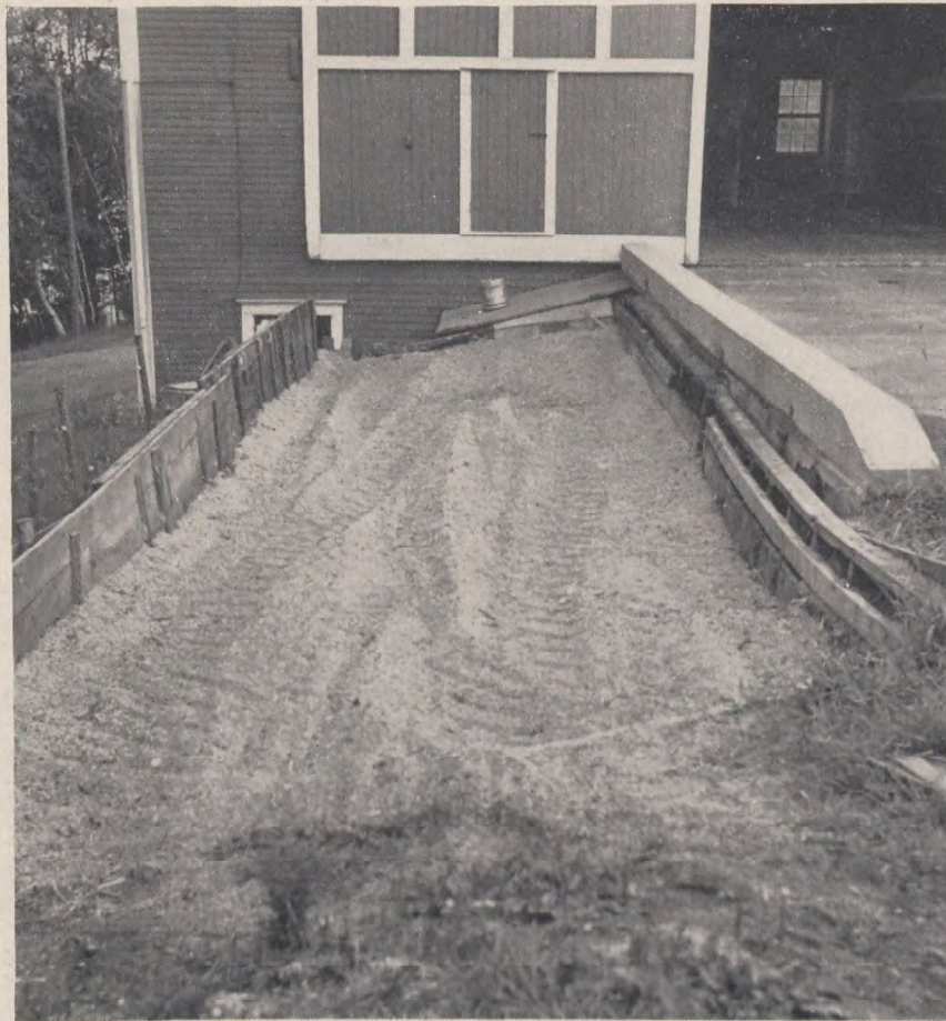
Figure 18. This trench silo at the Experimental Station, Kentville, is filled with grass silage packed down with a tractor, and covered with a layer of sawdust.
