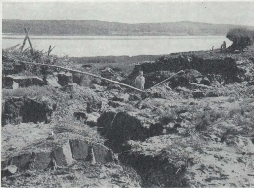
FIG. 19.—Tide has broken through dyke. Note the deep gully cut by receding tides. These gullies may run from 10 to 15 feet in depth.
