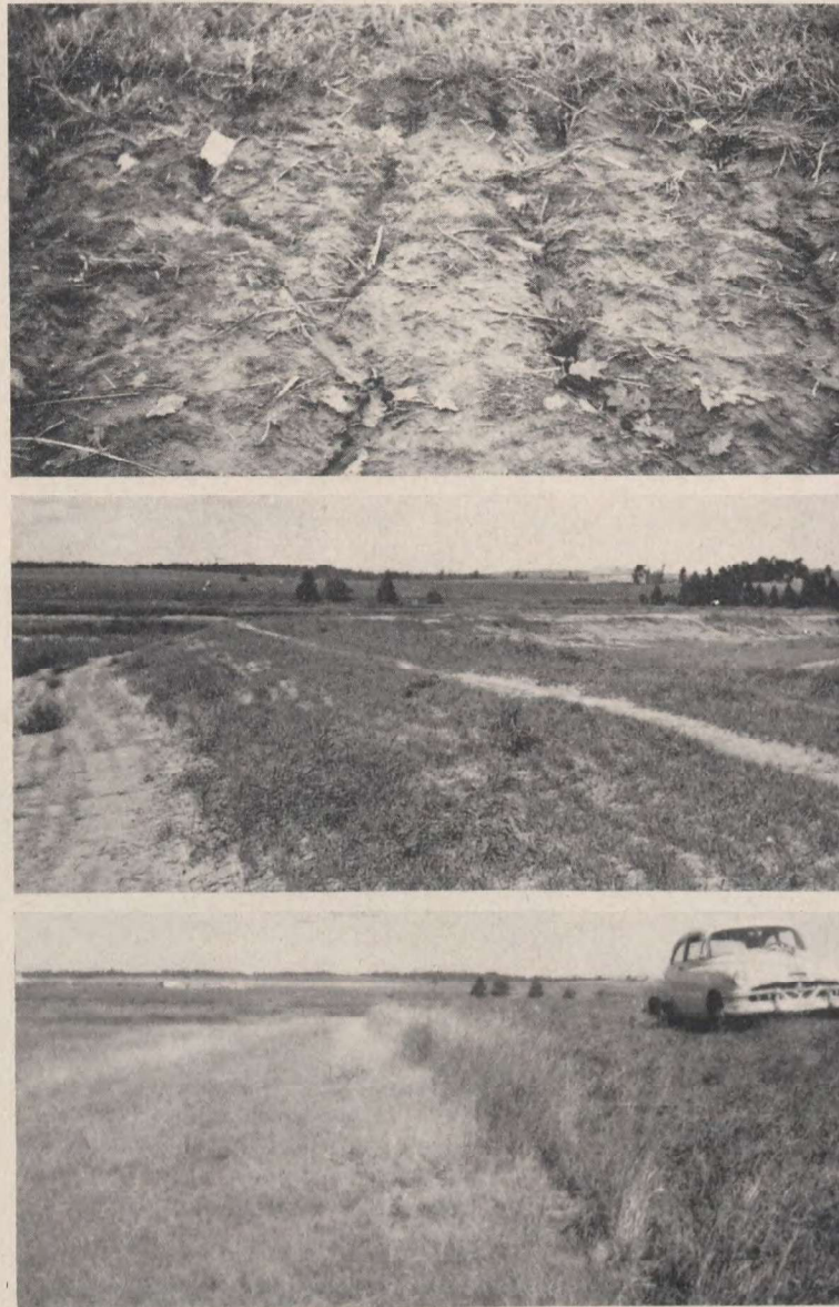
FIGURE 11. Certain varieties of grass can retard dyke erosion. Upper: Erosion starting on unprotected toe of dyke. Centre: Dyke seeded in 1951 with species lacking salt tolerance, growth has terminated at high-tide mark. Lower: Same area as in Upper protected by growth of Puccinellia maritima , a salt-tolerant species.
