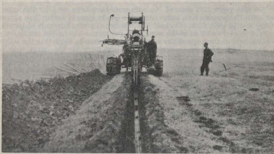
Experimental Station, Cap Rouge, Que. The draining machine at work. Drainage is very important but also very costly.
