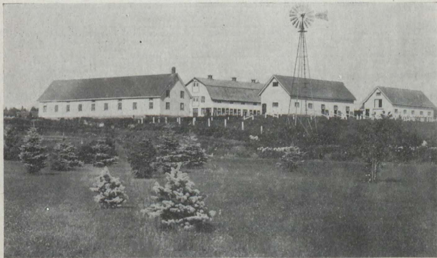
Implement shed, dairy barn, sheep barn and piggery at the Lennoxville Station.
