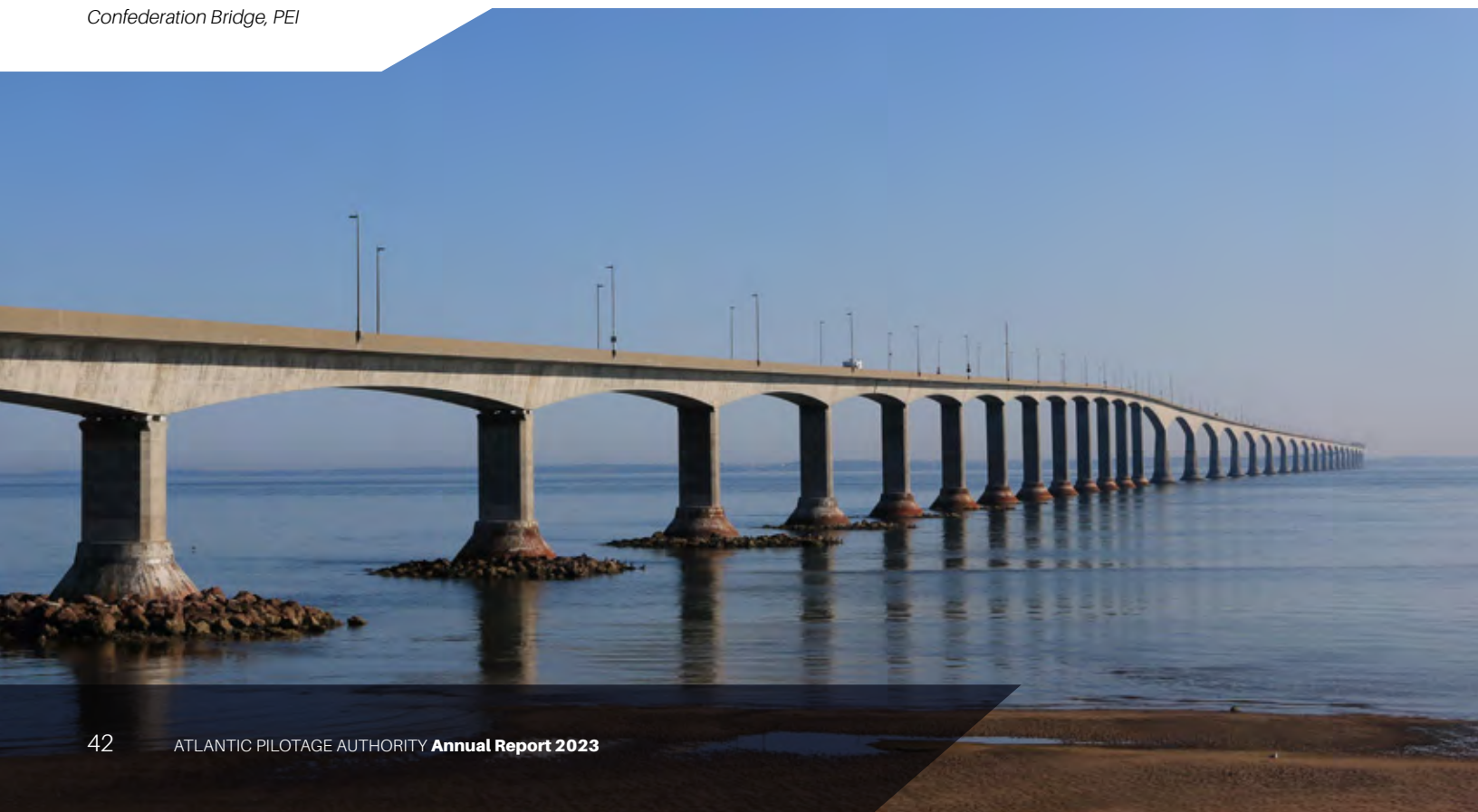
Confederation Bridge, PEI
