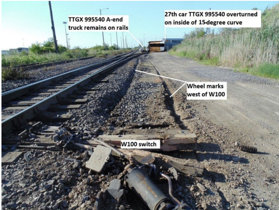
Figure 6. View southward from the W100 switch (Source: TSB)
