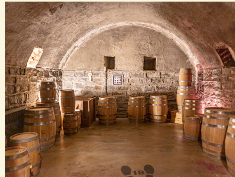
Interior of Martello Tower 1
