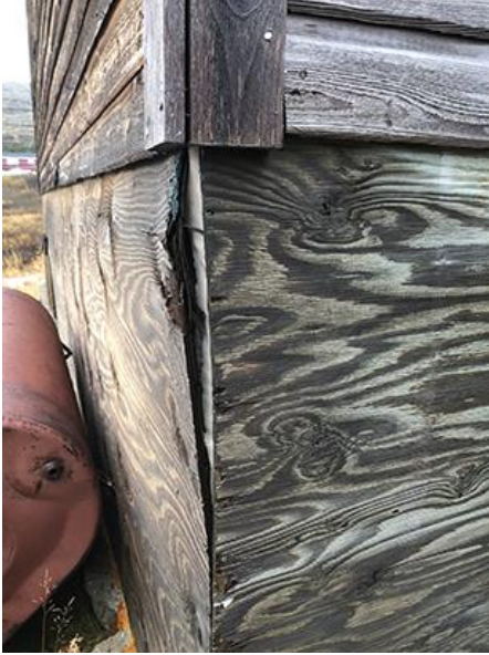
Bowed and water stained exposed wood foundations are a common sight in Nunatsiavut communities.
