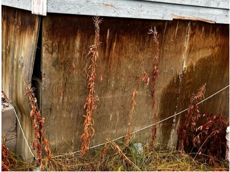
Bowed and water stained exposed wood foundations are a common sight in Nunatsiavut communities.
