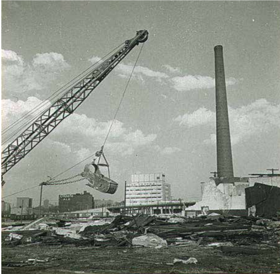
Figure 3 LeBreton Flats clearance and demolition.
