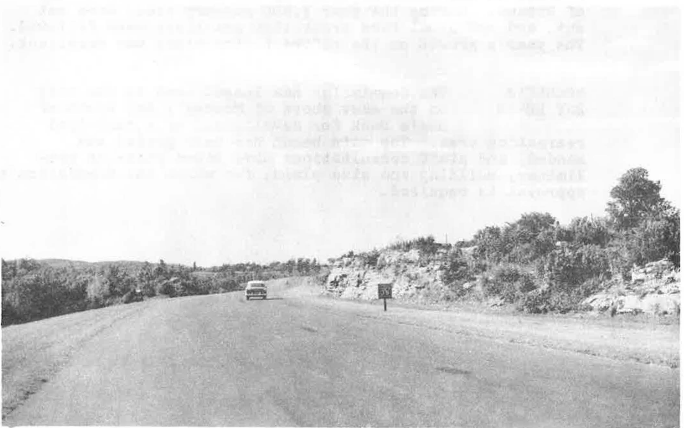
Top, Colonel By Drive, along the east bank of the Rideau Canal, Ottawa. Bottom, Lac des Fées Parkway, from near Blvd Taché to Blvd Gamelin, Hull.
