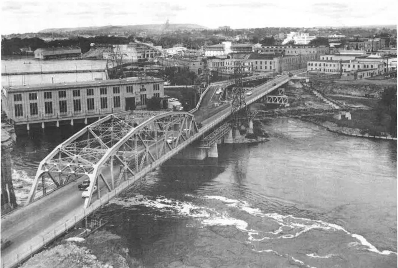
The improved Hull approach to the Chaudière Bridges over the Ottawa The right lane of the divided roadway section is on the new steel span
