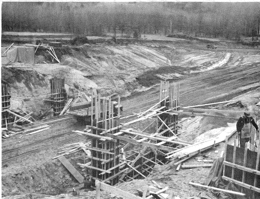
Kingsmere Road Overpass under construction.
