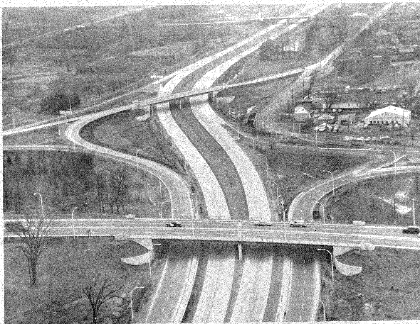
The Queensway, a Municipal, Provincial, Federal and NCC co-operative project which will give Ottawa a high-speed east-west thruway built partly on former CNR rights-of-way. Photo shows the Alta Vista, "M" Avenue and Tremblay Road overpasses.
