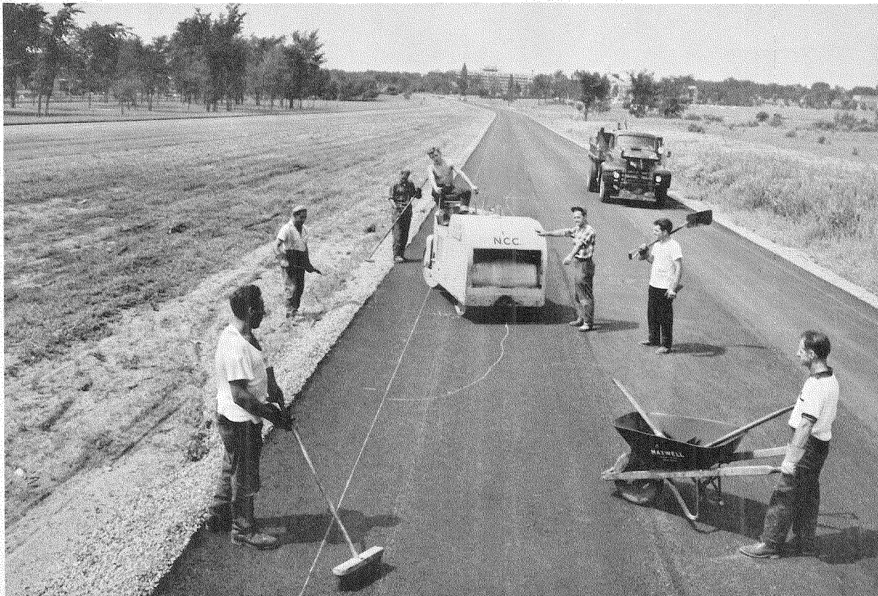
Second strip of Eastern Parkway being completed by NCC workers.
