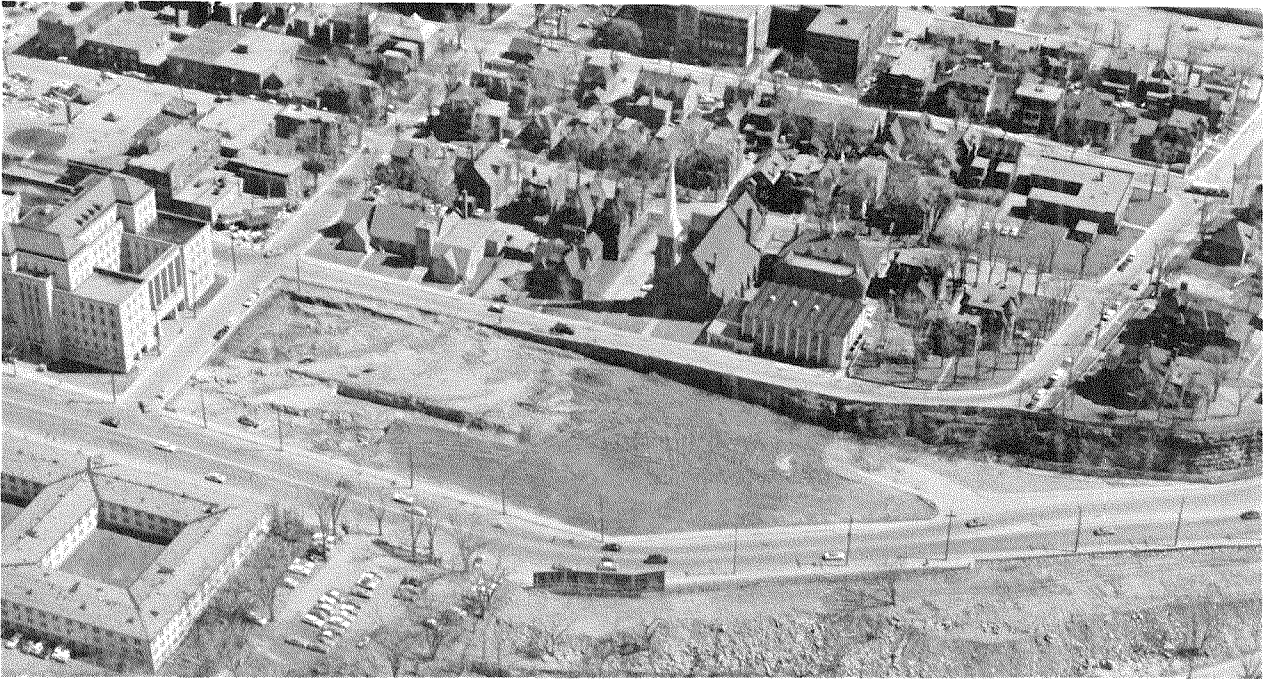
Garden of the Provinces in construction.
