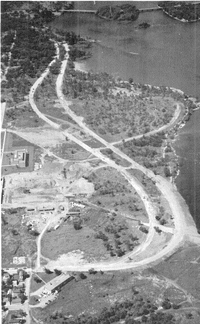
Aerial view of Ottawa River Parkway now in construction.
