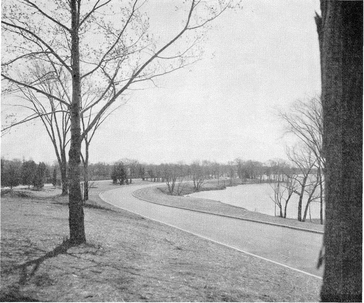
Ottawa River Parkway extension to Woodroffe Avenue.
