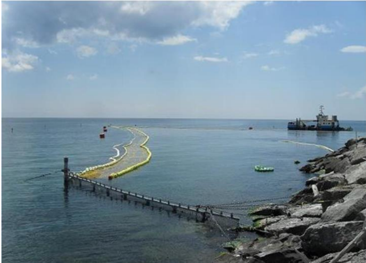
Figure 2.2: Ontario Power Generation’s fish diversion system, a mitigation structure to reduce the biomass of fish impingement [10]
