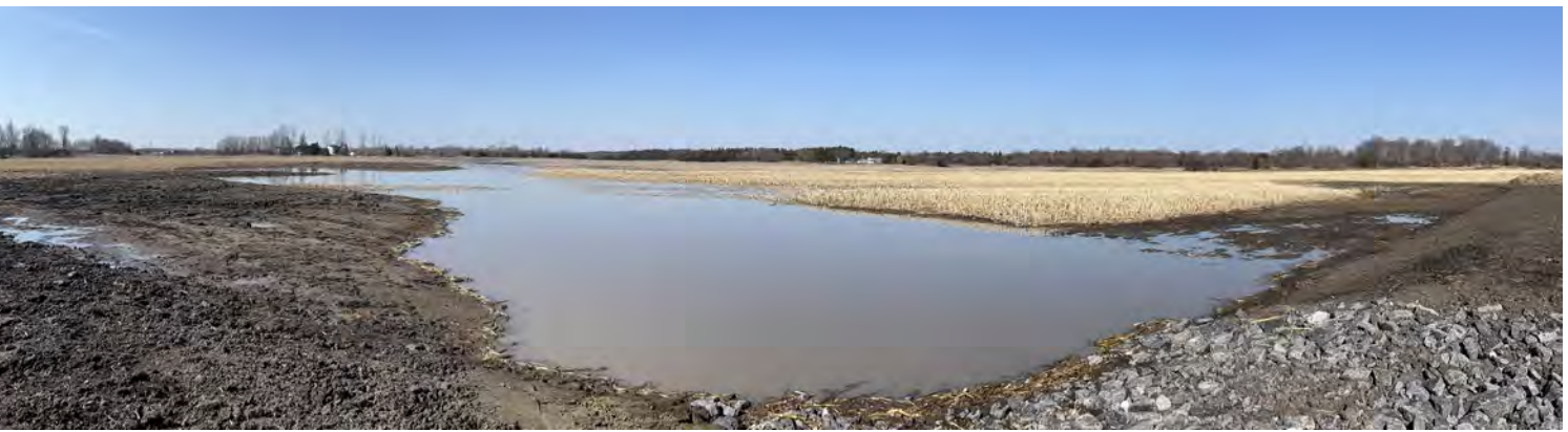
The earthen berm and spillway, with riprap to prevent erosion.
