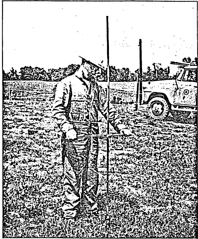
Soil Test Probe being used to determine class of soil
