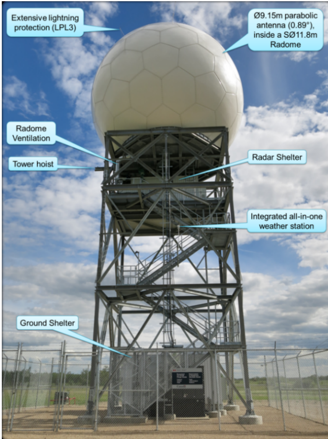
Photo of the new radar design. All ECCC radars are carbon-copies of each other – same technology, same design. The only difference between radars is the height of the tower and the specific frequency assigned to the radar.
