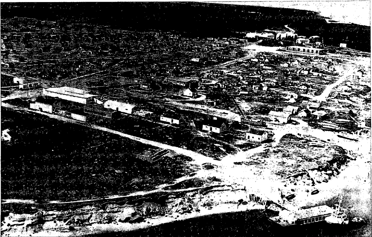
Bank Erosion Fort George, Quebec
