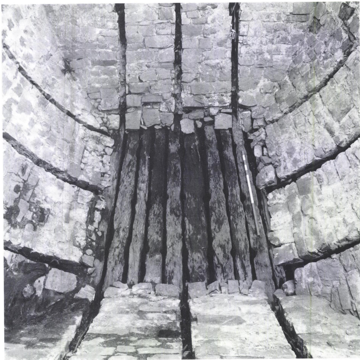
2.9 The platform used to support the ice.
