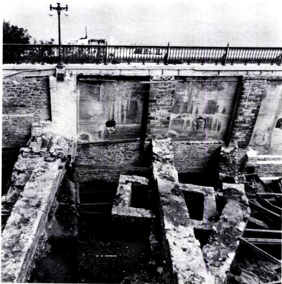
3.13 General view of the remains of the greenhouse built over the earlier ruins of Fort Saint-Louis and of a building of unknown function.
