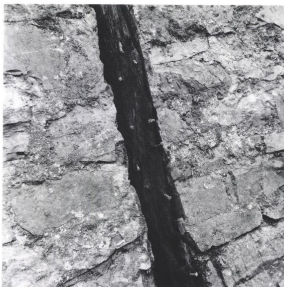
2.12 The forged nails used to attach the wooden facing were still visible. (Canadian Parks Service, photo: Michel Élie; 38G86R32X-8)
