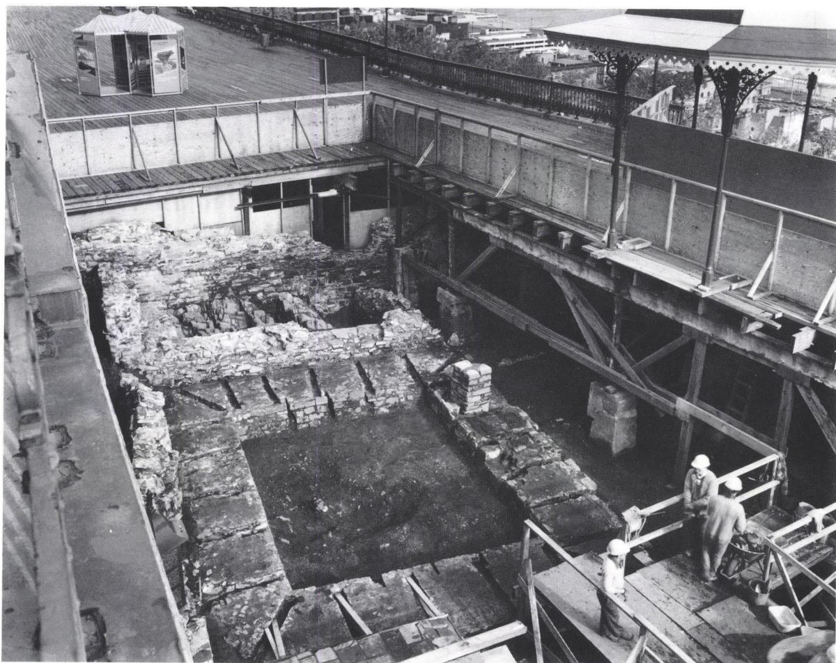
2.3 The icehouse found under the Dufferin Terrace, during the course of the excavation. (Canadian Parks Service, photo: Michel Élie; 38G85R103X-11)
