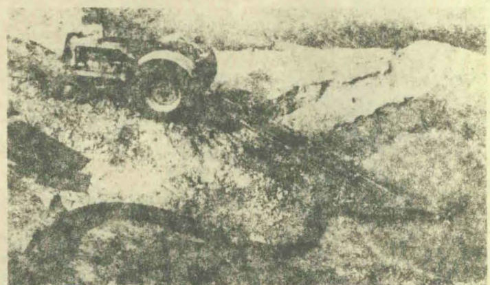
DEWATERING GRAVEL PIT WITH LONG HITCH MODEL
