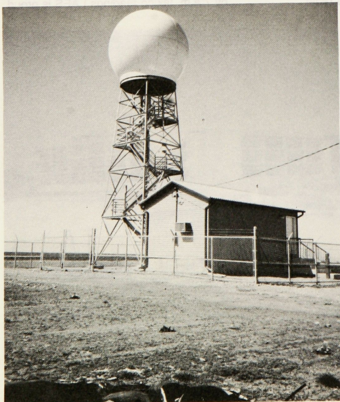
Calgary Radar Station, Vulcan, Alberta.
