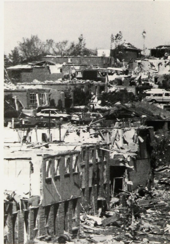
Townhouse complex in Barrie, Ontario, devastated by tornado in May 1985
