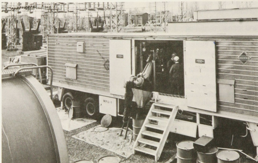
An Ontario Hydro mobile PCB decontamination unit.
