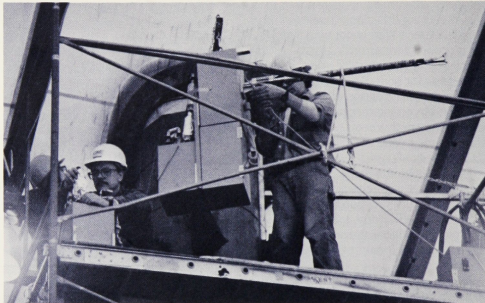
Stack emissions were regularly checked to make sure that incineration was effective.
