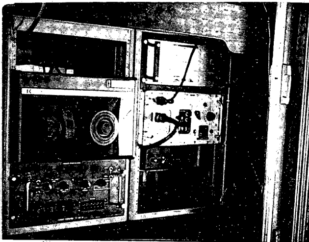
Equipment installation in VERITY.
