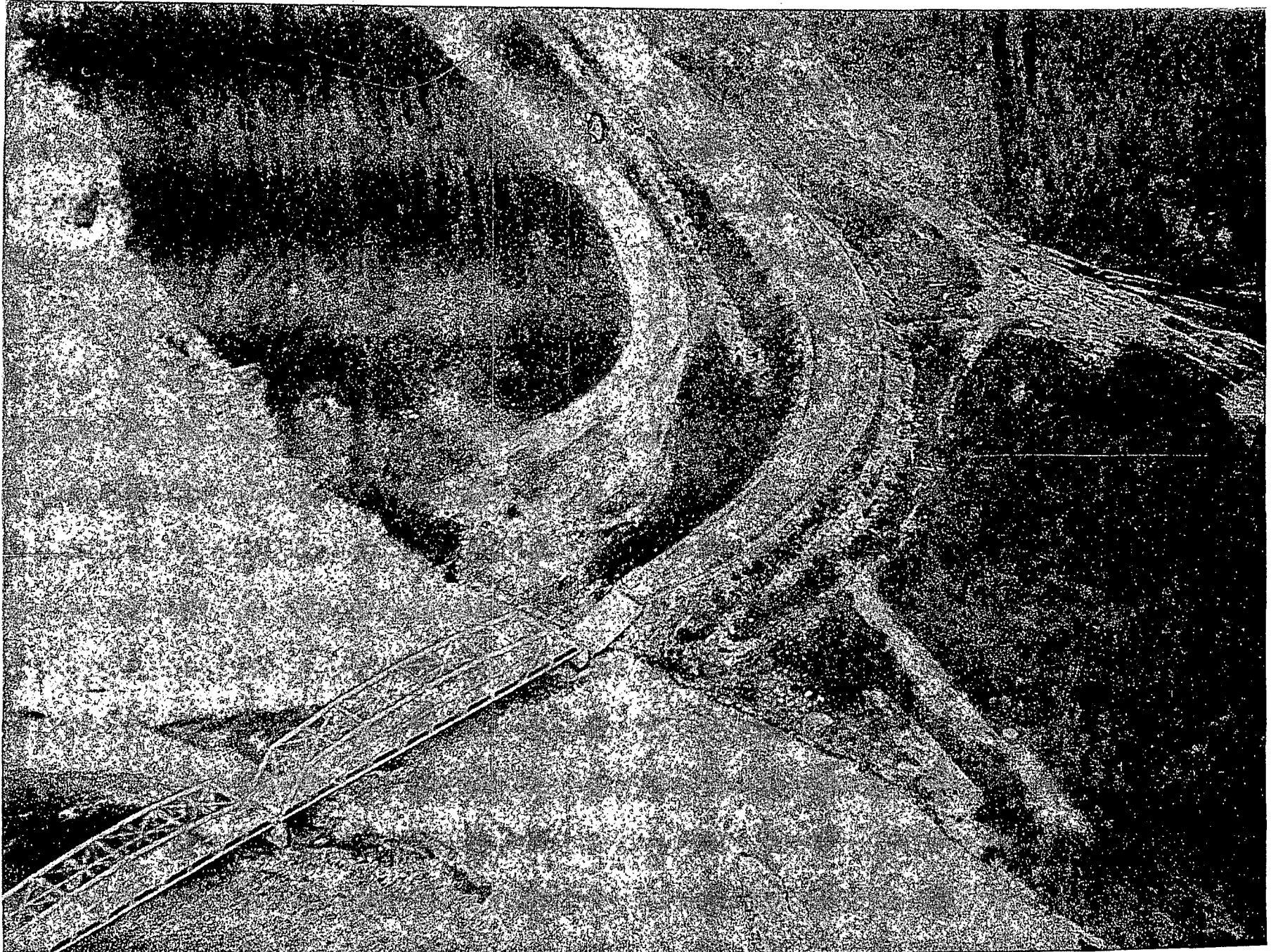
Figure 13 Washed-out bridge approach at Racing River, British Columbia, July, 1974 (Whitehorse Star Photo)
