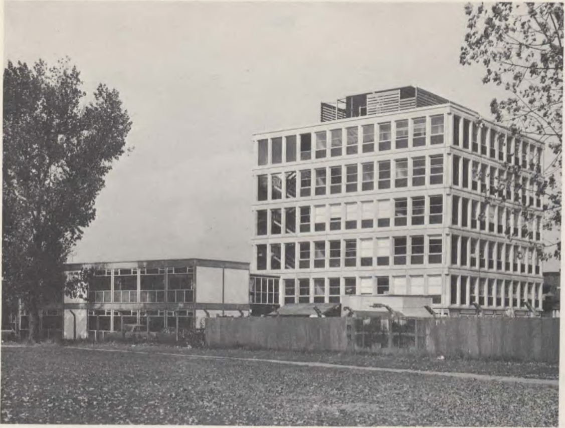
Six storey office building erected in the Laingwall system at Boreham Wood, Hertfordshire, for the Research and Development division of John Laing Construction Limited.
