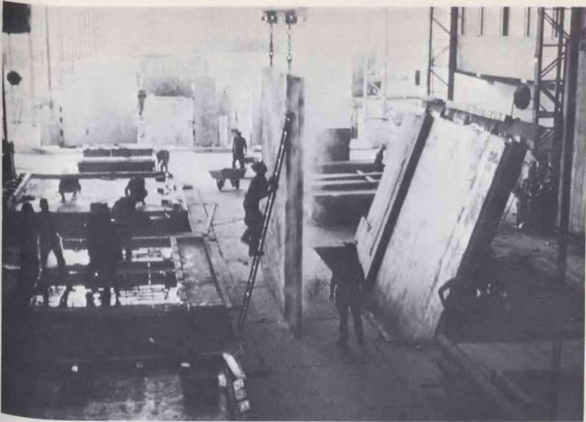
Cured panel removed from casting table.
