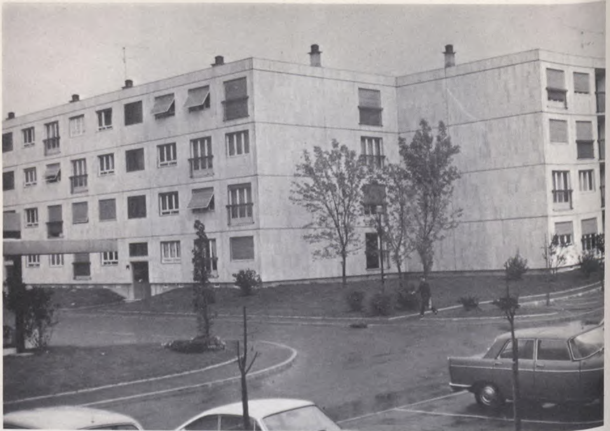
Luxury apartment near Paris. Travertine was used as facing material on panels.
