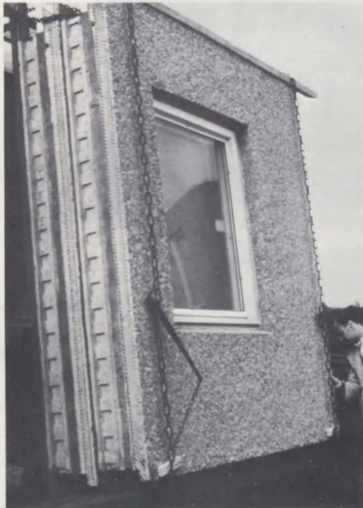
Precast façade panels manufactured by Swedish licensee of Jespersen system for apartment project near Malmö.
