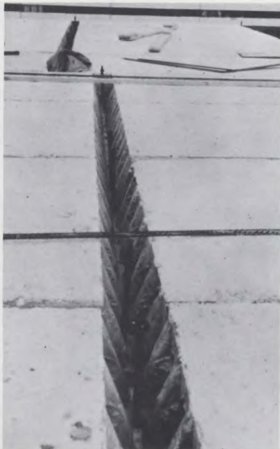
Apartment project near Malmö - showing floor elements installed.
