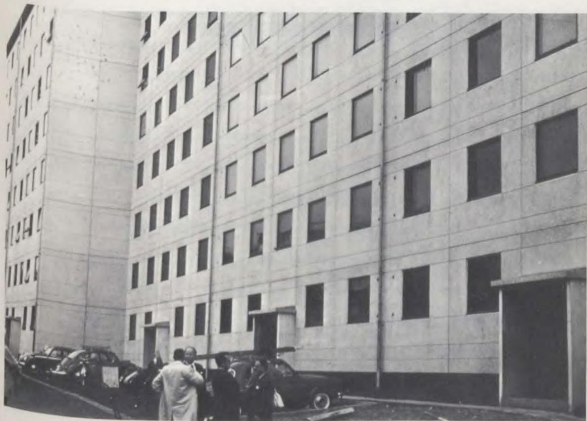
Apartment building under construction in Copenhagen.
