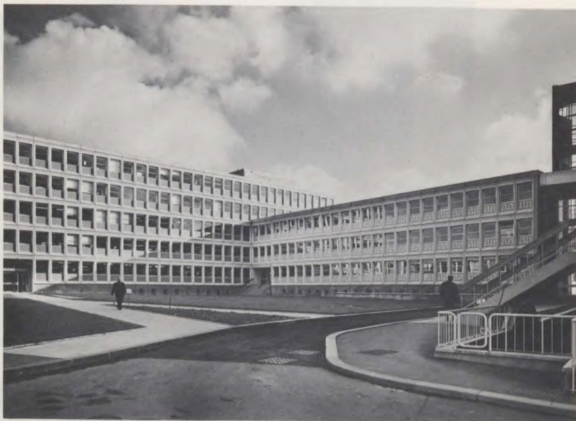
Head offices of John Laing and Son Limited at Mill Hill, London, N.W.7, erected in the Laingwall system of industrialized building.
