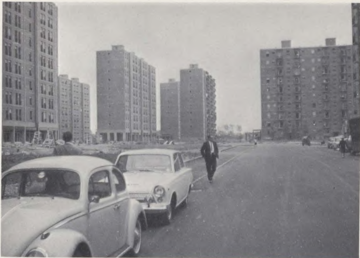
Low rent apartment project near Milano.
