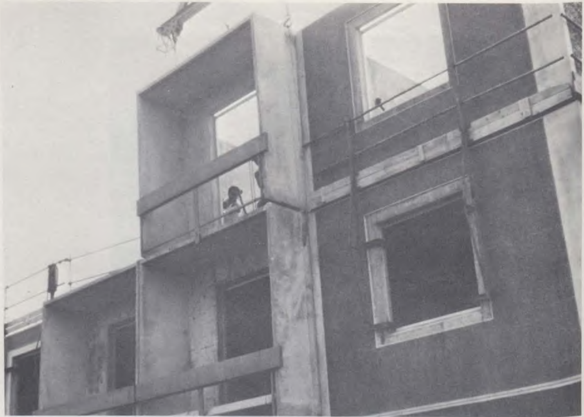
Balcony being erected.
