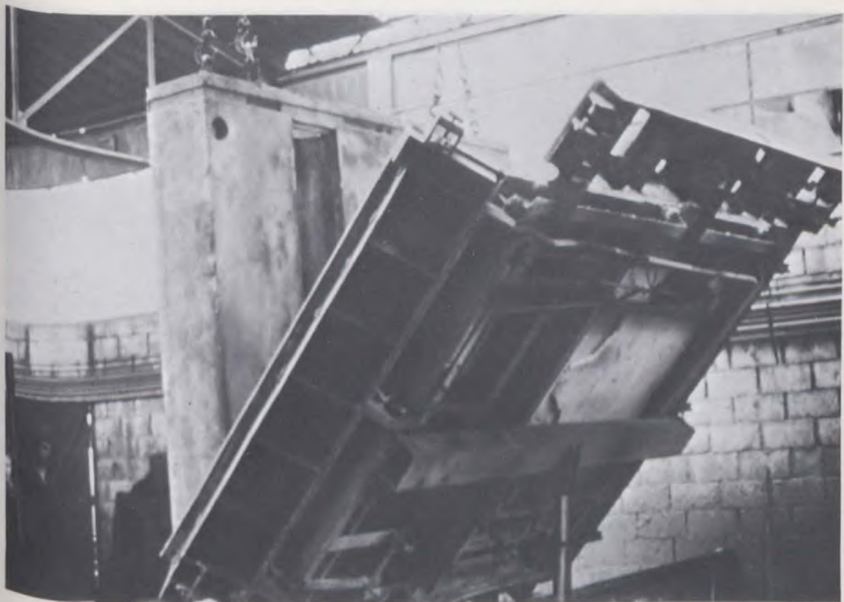
Demoulding of a functional unit.
