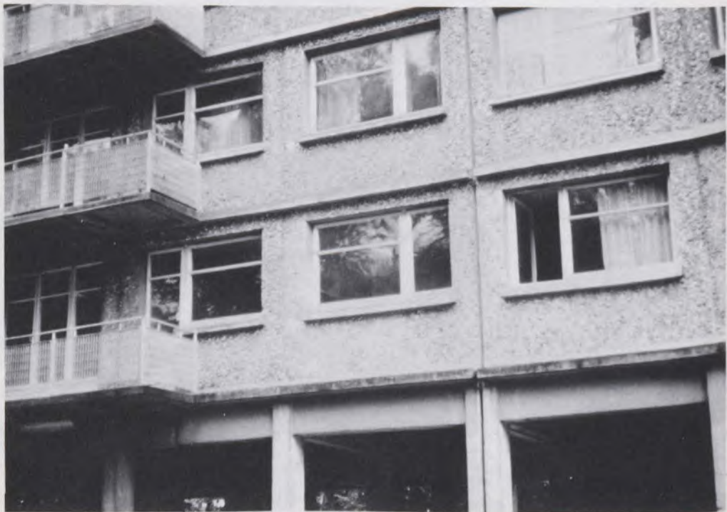
SHAPE HQ near Paris - built 20 years ago. The quality and condition of the building is still excellent.
