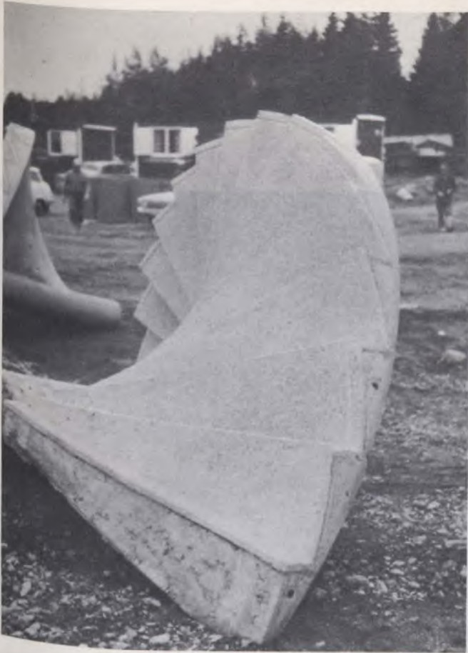
Precast circular stairs.
