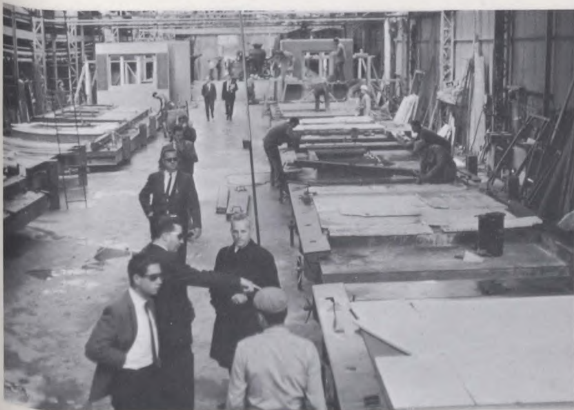
Horizontal façade moulds.
