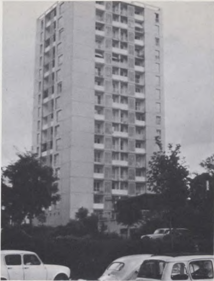
16 storey low rent apartment building in Paris.
