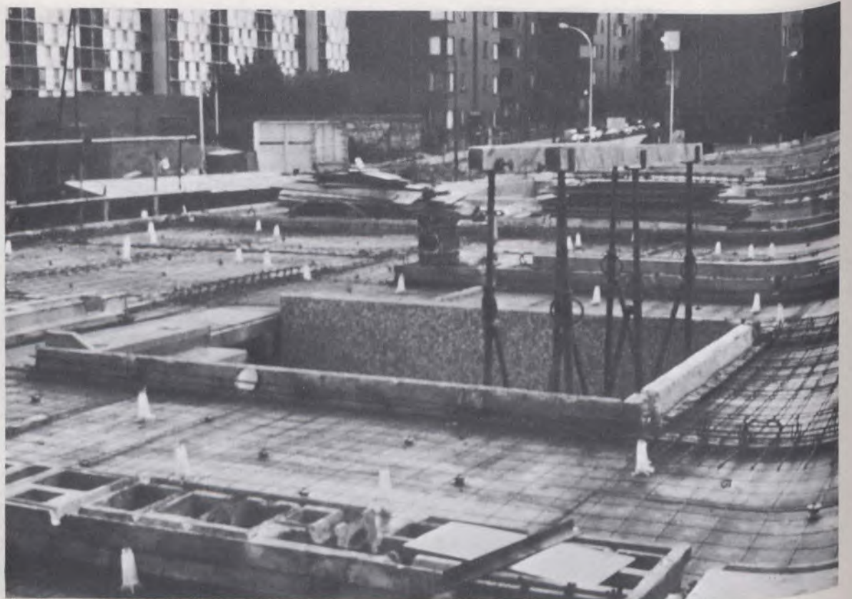
Floors are poured in situ on precut formwork.
