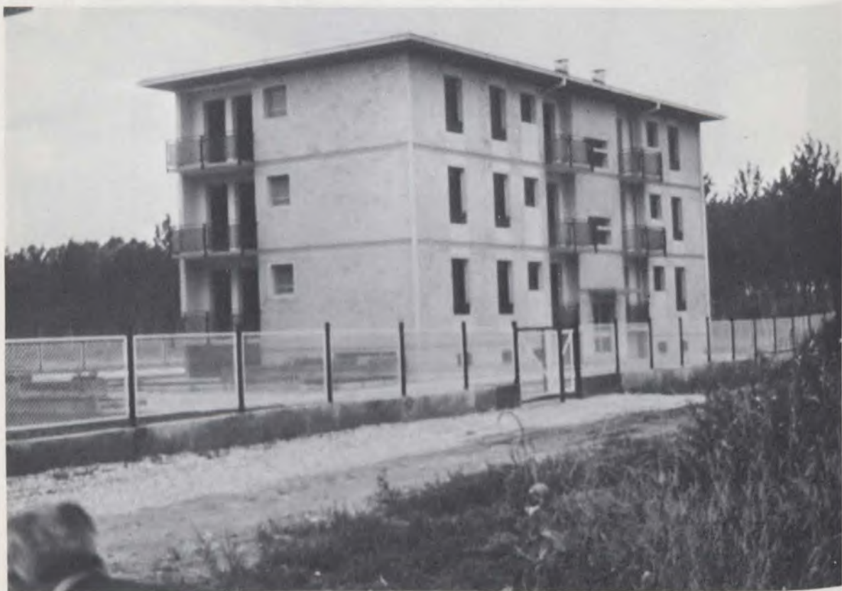
Experimental apartment made of brick panels precast in plant.
