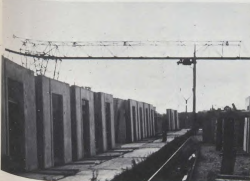
Wall elements with door openings.
