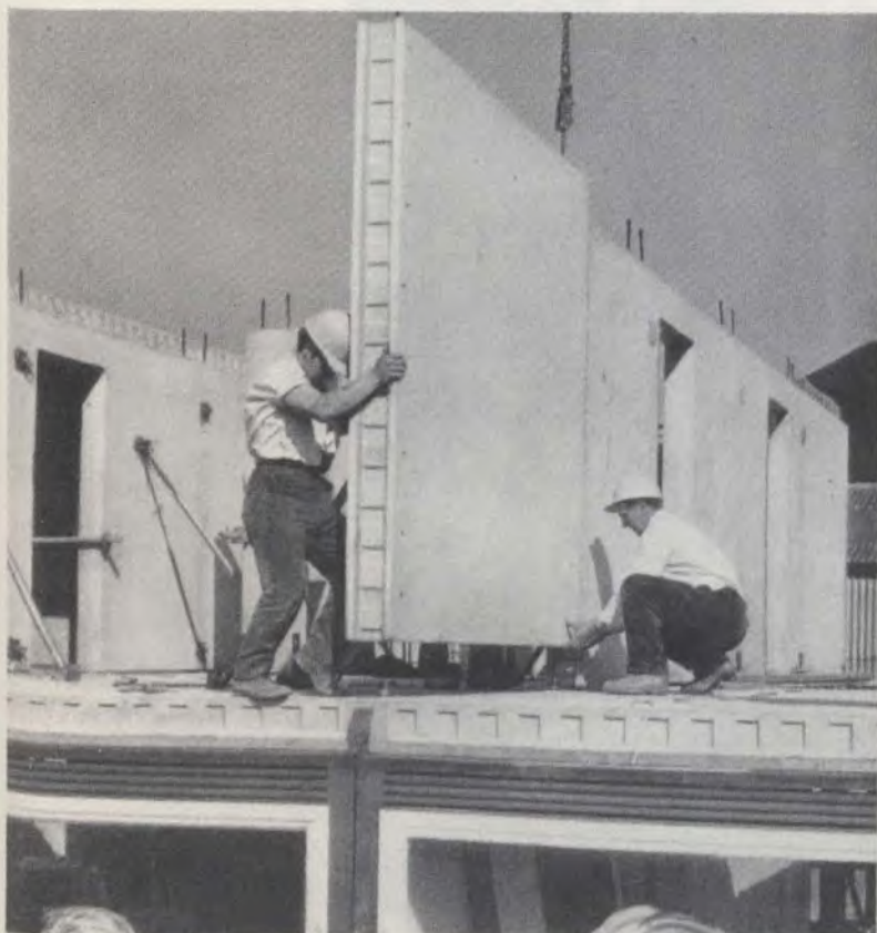
Placing of wall elements.
