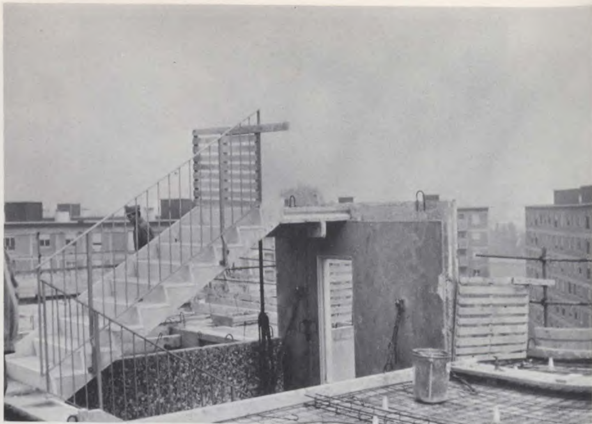
Installation of stairs.
