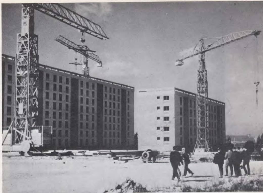
Large project under construction near Paris.
