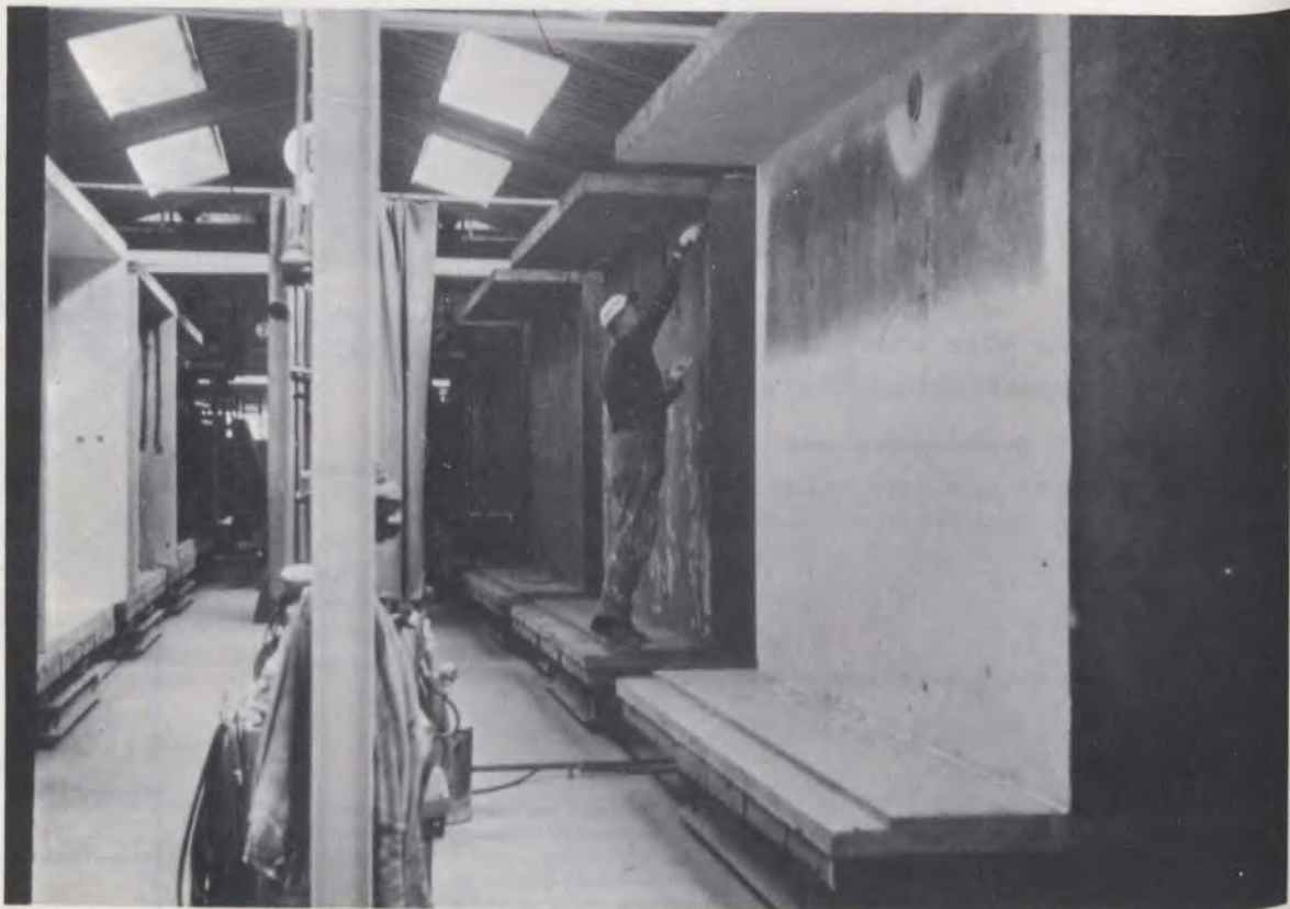
Workman executing minor repairs prior to painting.
