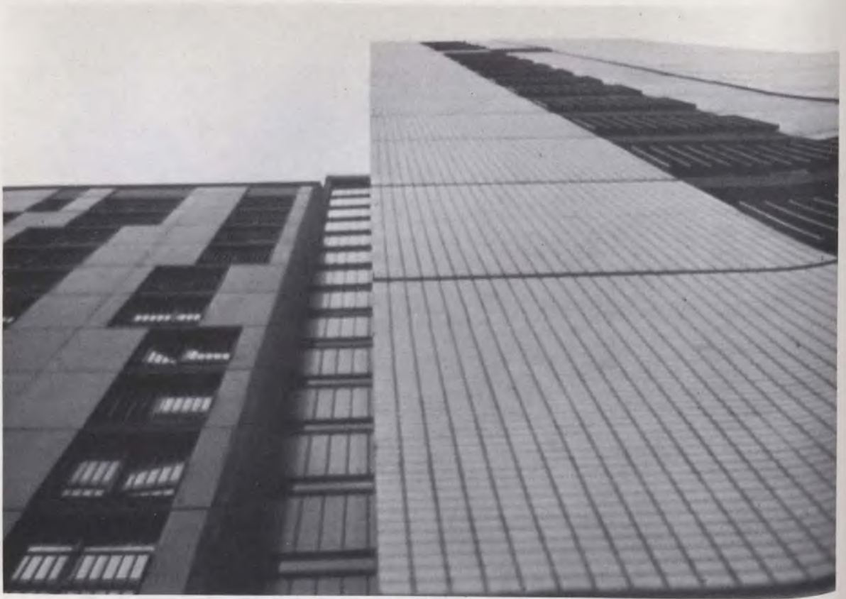
2" x 2" ceramic tiles on façade panels.
