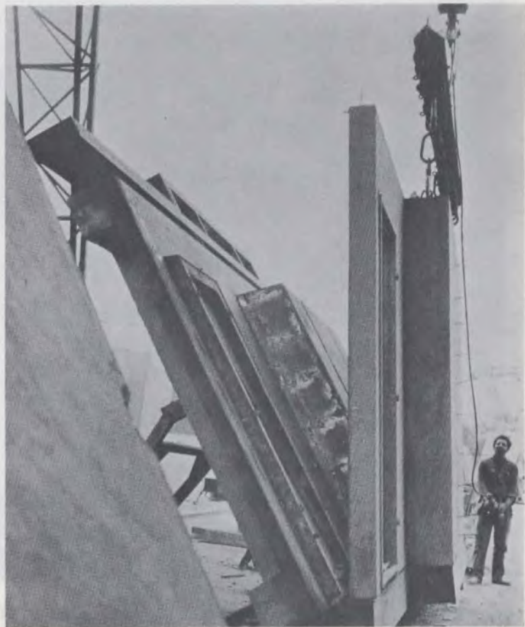
Precasting moulds.
