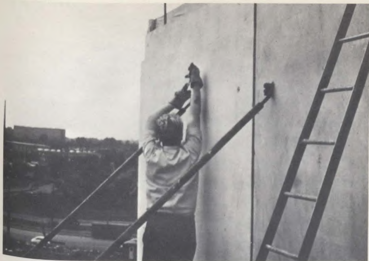
Securing façade panel.
