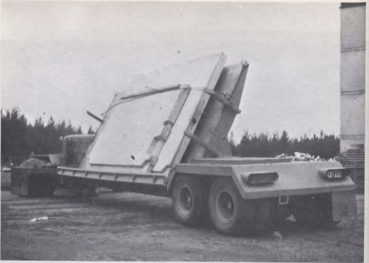
Special trucks equipped with hydraulic tilting platform.
