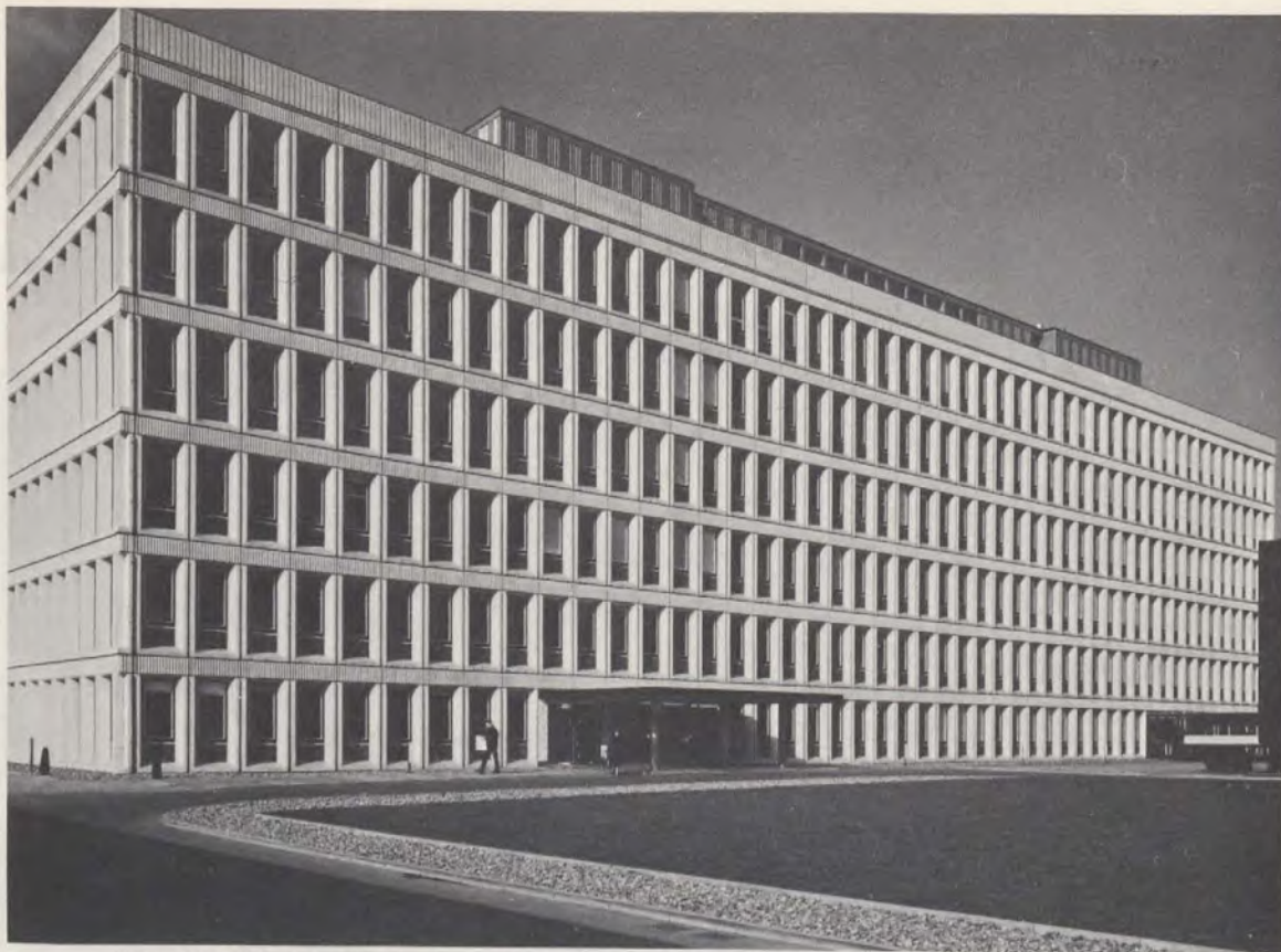
The North Western Gas Board's new headquarters at Altrincham, Cheshire, erected in the Laingwall system of industrialized building.
