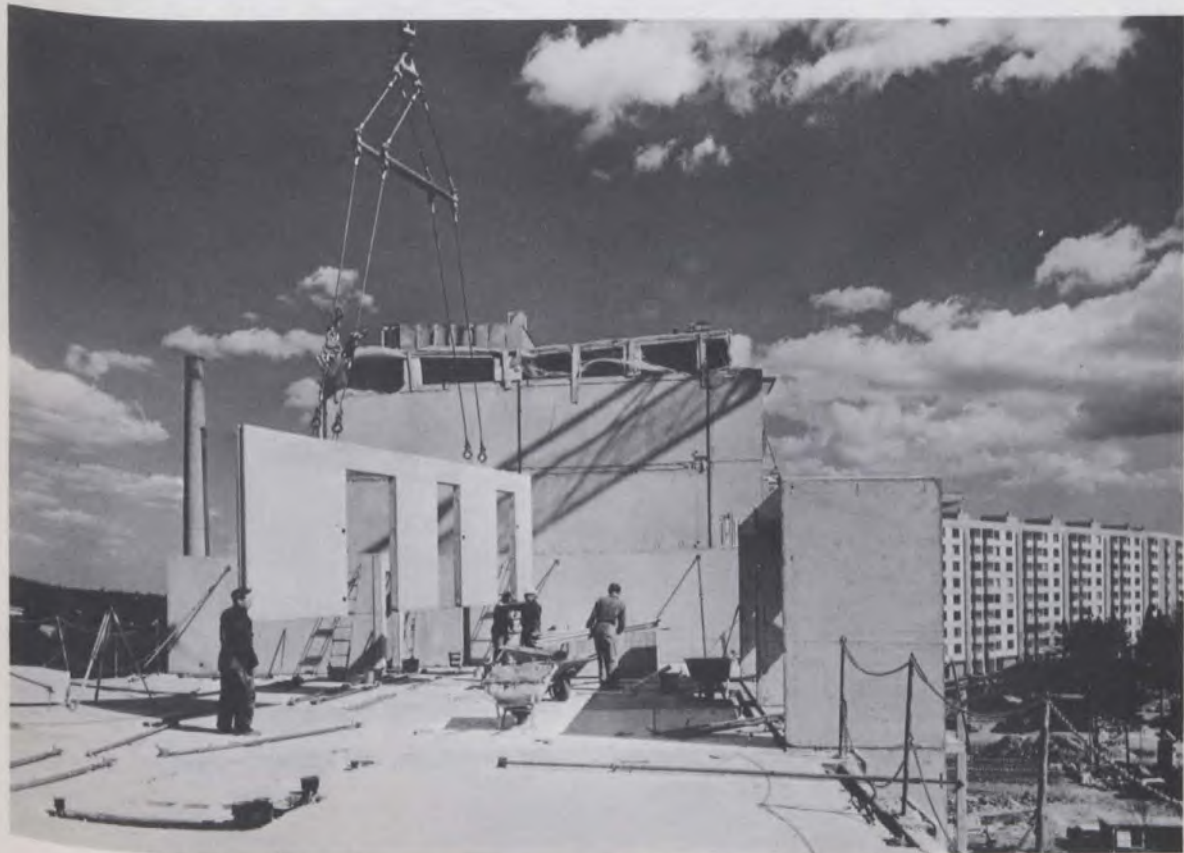
Sharne heavy system - inner wall element weighing 6 tons.
