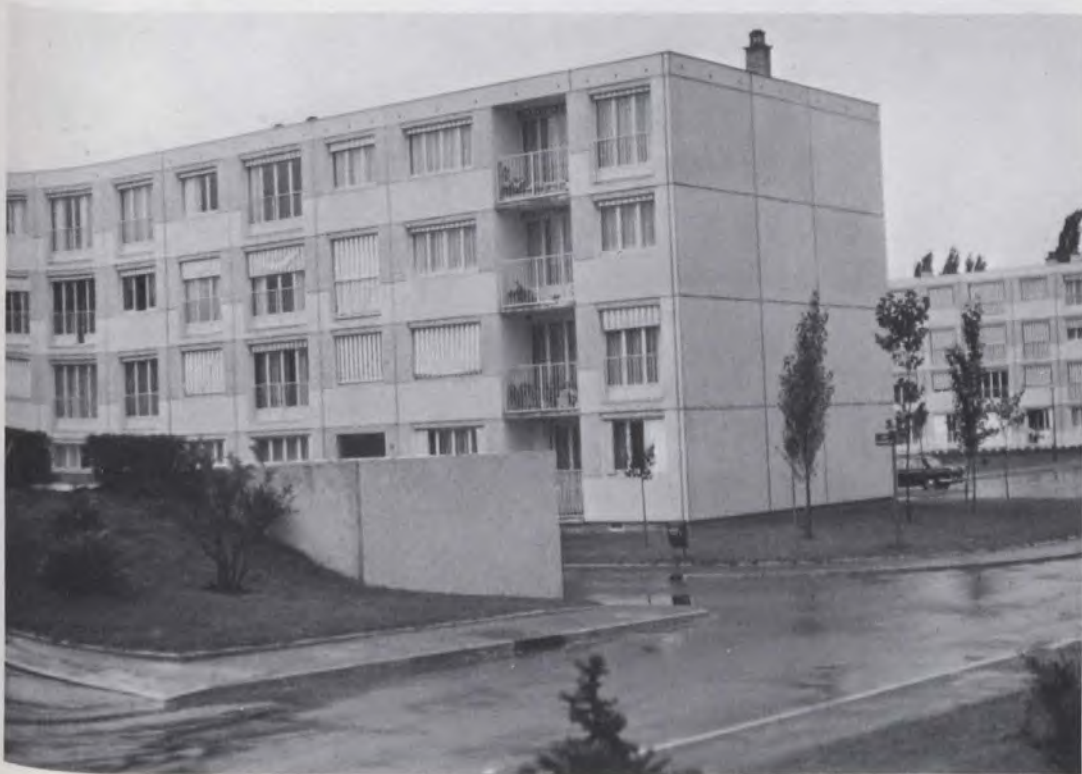
Medium rent apartment project.
