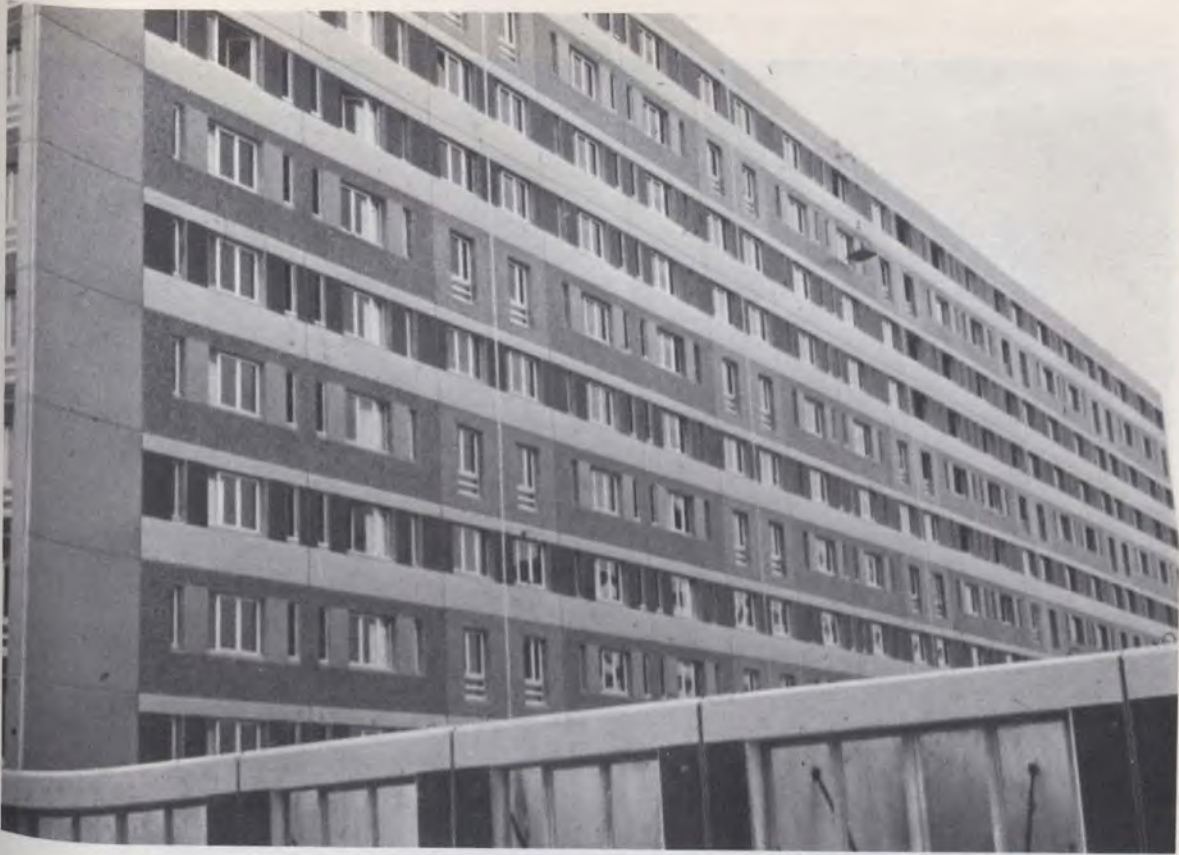
Low rent apartment project under construction near Paris.
