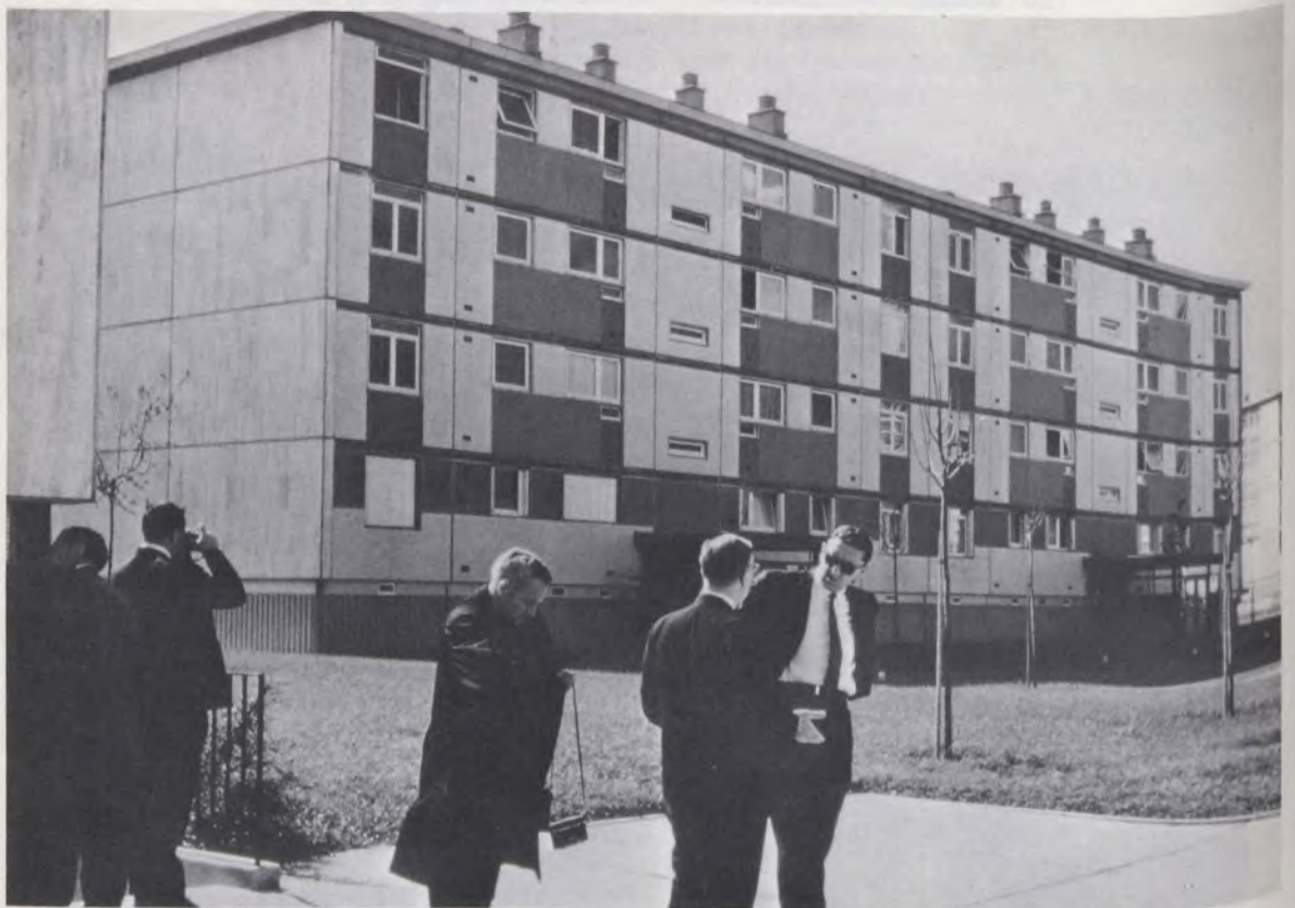
Medium rent apartment near Paris. Facing material used was Travertine and Slate.
