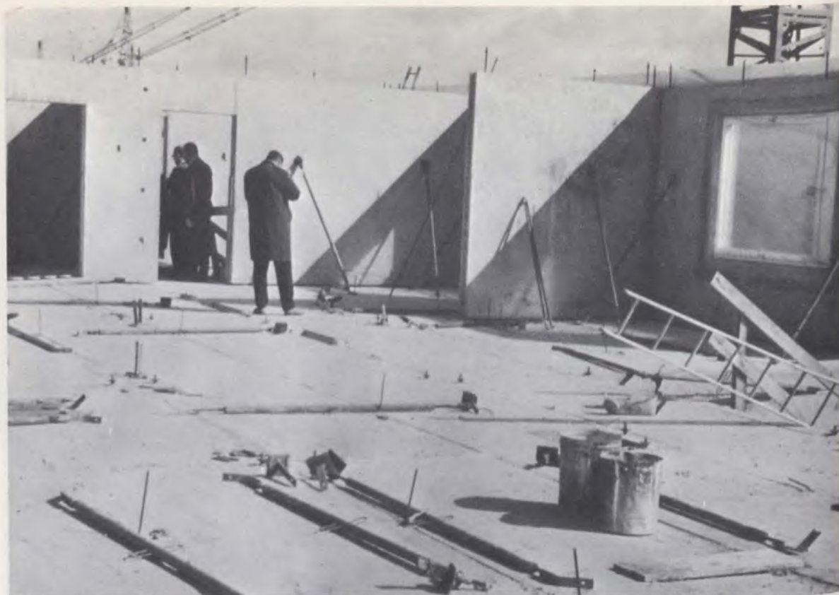
Apartment project near Malmö - showing wall and floor elements being erected.
