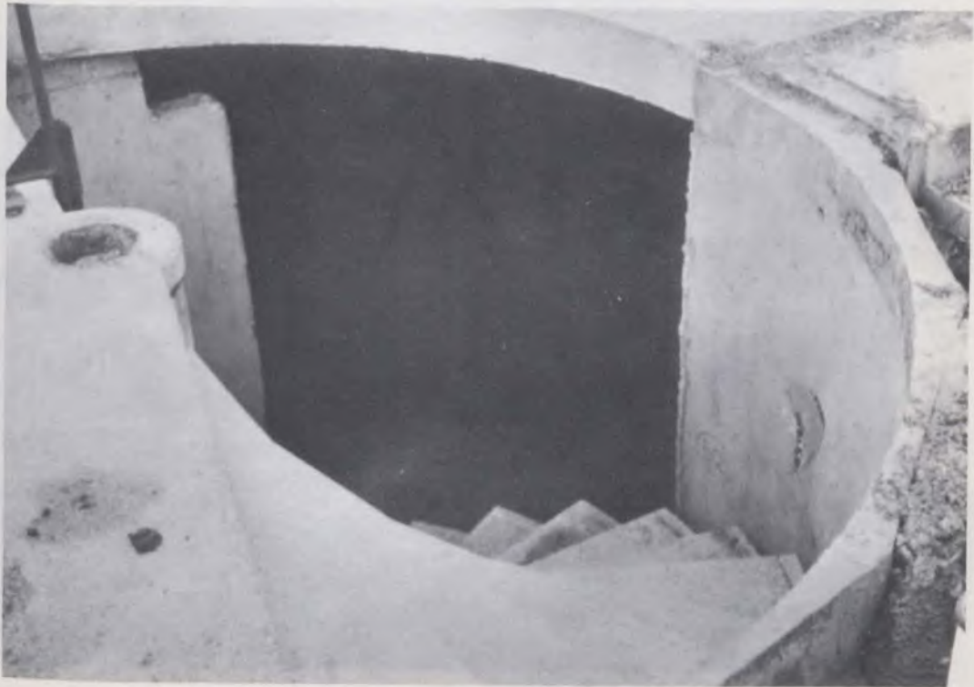
Precast circular stair installed.
