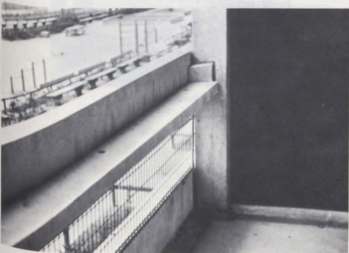
Gladsaxe - Detail of balcony construction.
