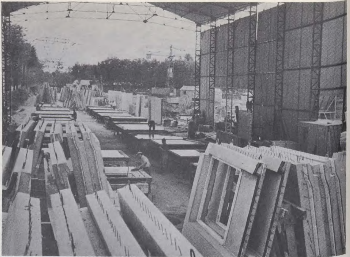
Precasting factory with a capacity of one apartment per day at Thais near Paris.
