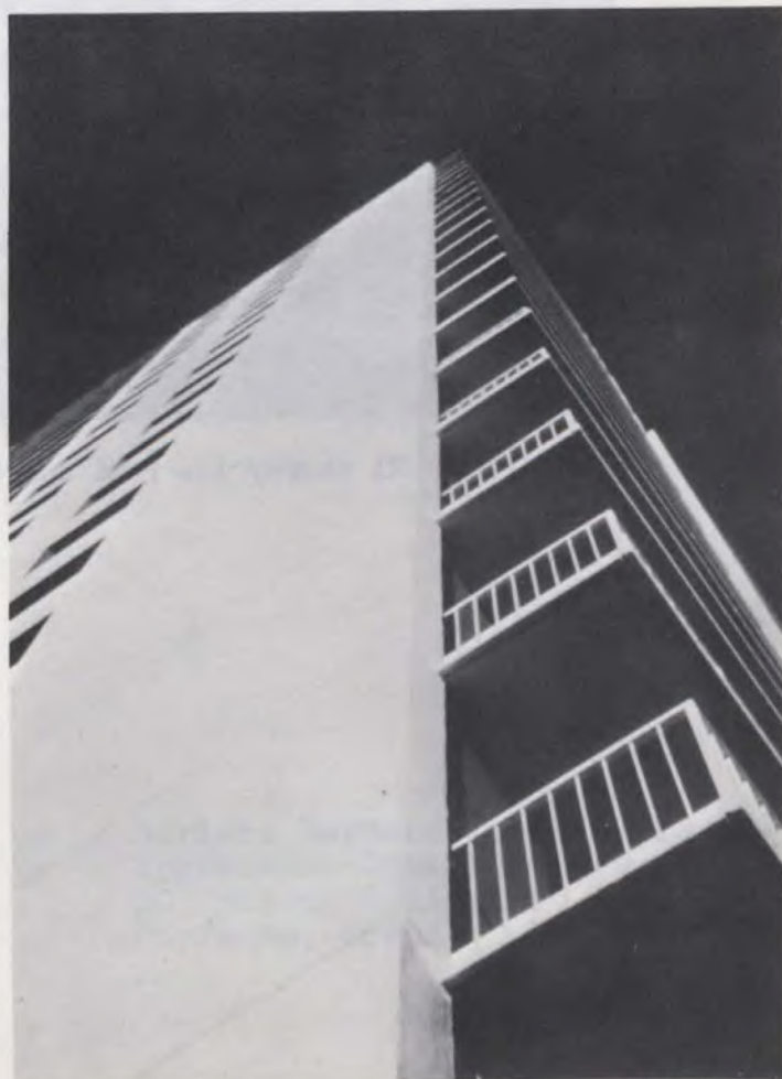
Low rent apartment building - high quality concrete panels.
