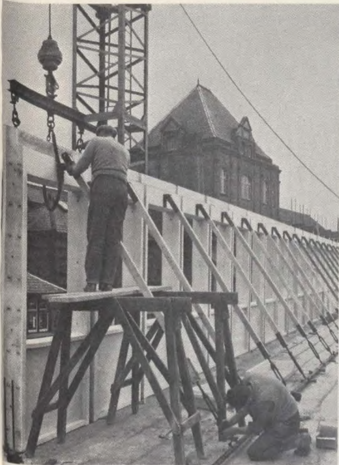
Precast floor units being placed, spanning between Laingwall units and spine beams running down centre of building.
