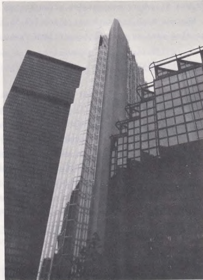
Figure 5: The Royal Bank Plaza, Toronto - Where Fly Ash was used in High-Strength Structural Concrete.
