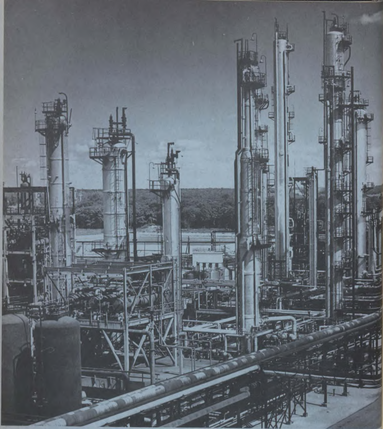
Hydrocarbon streams from neighboring oil refineries are piped into this feed preparation area at Polymer Corporation Limited at Sarnia, Ontario and treated for use in making synthetic rubber.
