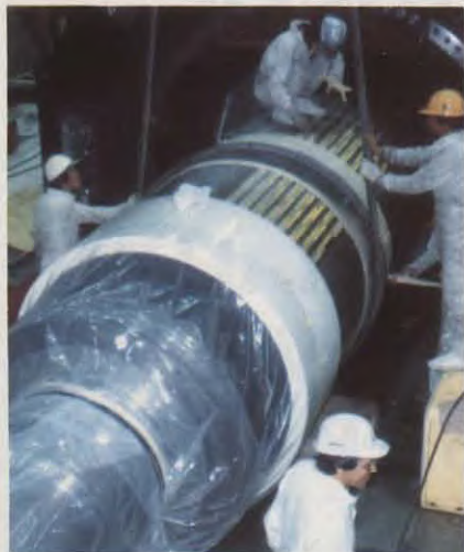
Installation of generator rotor at Wolsung Nuclear Generating Station – Korea
