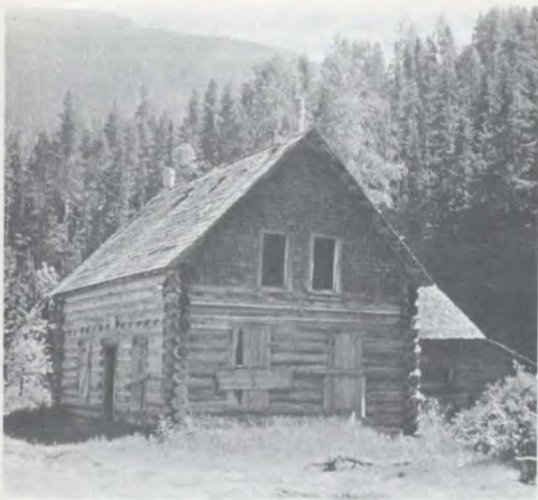
Figure 16. This old hotel at Kitsumkalum Lake, near Terrace, in British Columbia, is part of a system of trails, cabins, and other hotels associated with the anticipated overland telegraph from New York to Europe via Alaska and Siberia. Portions were built and operated, but the first trans-Atlantic cable stopped construction. Most of the buildings, as well as the trail, have disappeared, but the remains are significant as focal points for historical interpretation and display. The small land unit is designated 5U HV.
