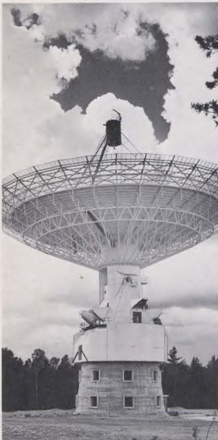
Canadian National Research Council's giant radio telescope at Lake Traverse, Algonquin Provincial Park, Ontario, has a 150-foot diameter parabolic reflector.
