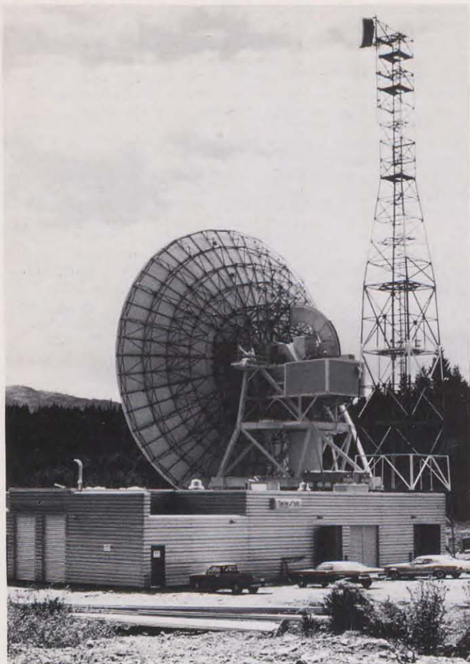
Canada's vast communications system includes integrated satellite and microwave networks which, when complete, will cover the entire nation. Shown are a satellite ground relay station and a microwave tower.
