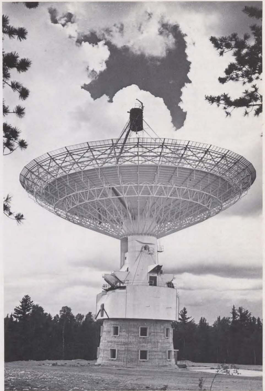
Canadian National Research Council's giant radio telescope at Lake Traverse, Algonquin Provincial Park, Ontario, has a 150-foot (45-metre) diameter parabolic reflector.
