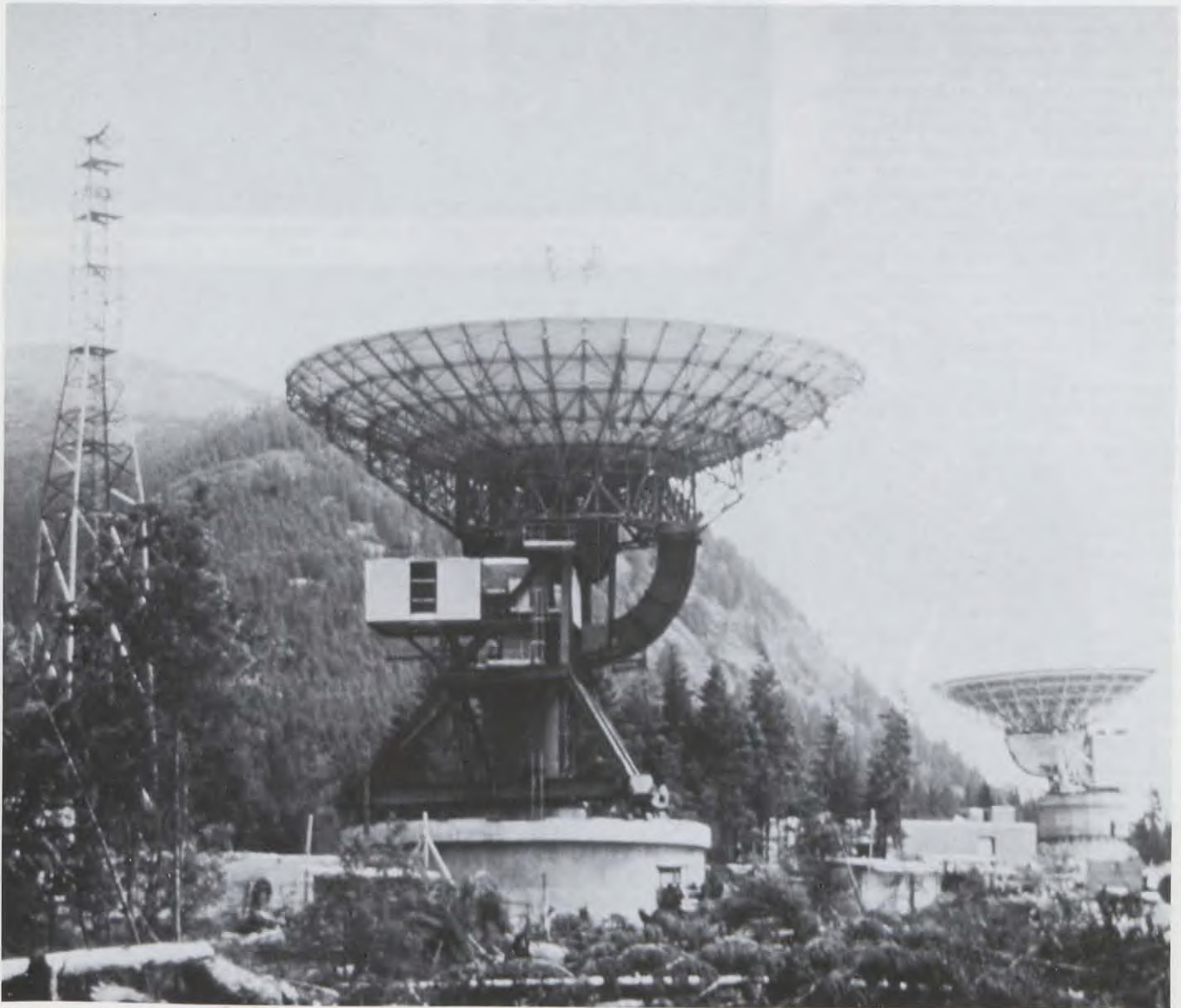
Teleglobe Canada and Telesat Canada large satellite earth stations at Lake Cowichan for international and domestic services.
